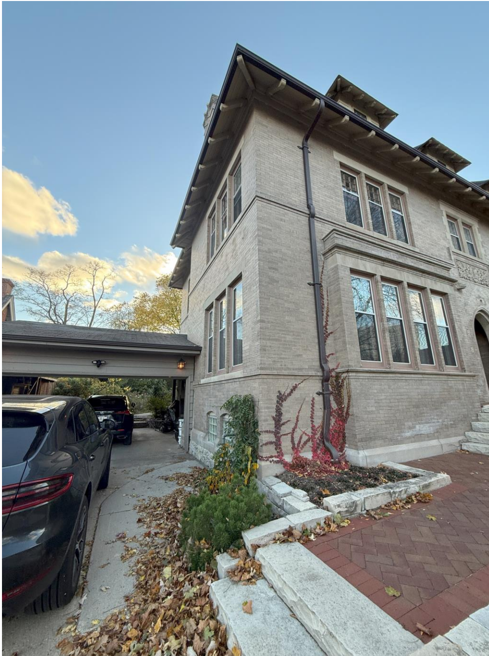
Garage at left to be demolished.
