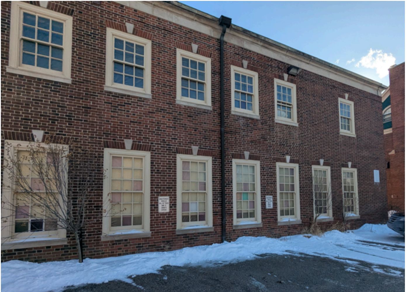
Exterior Overview of building
