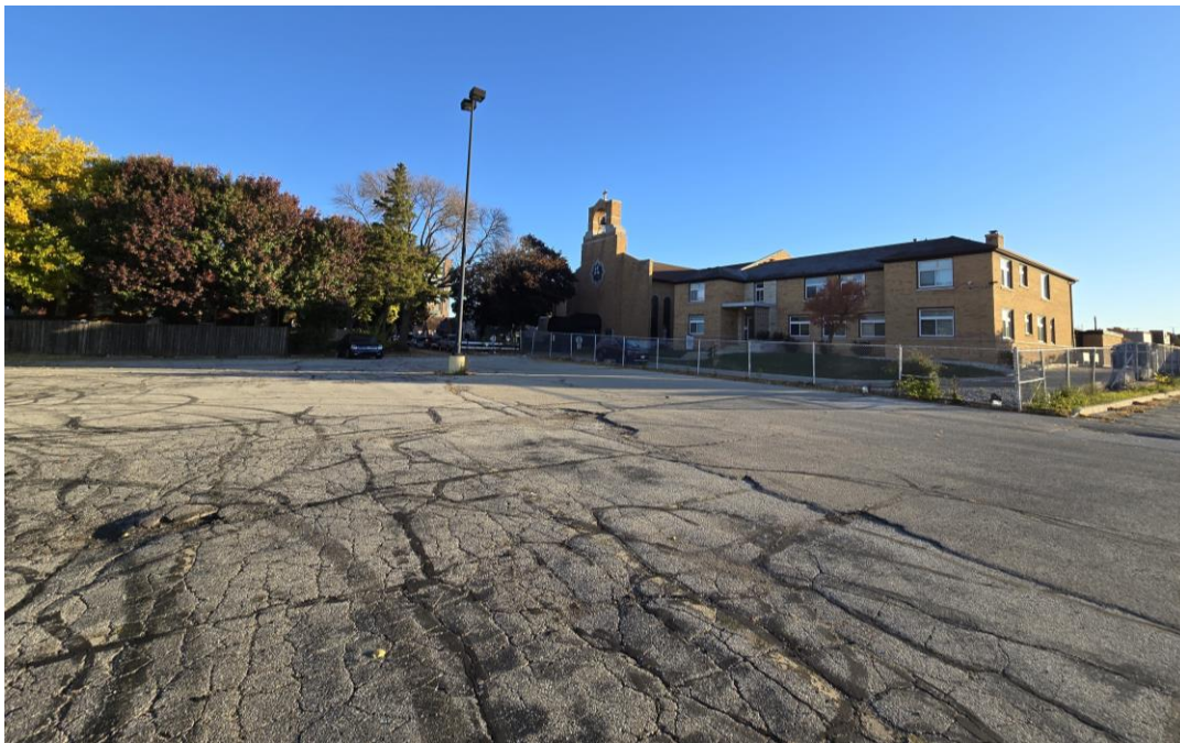
Image 6: view of north side of lot, looking north
