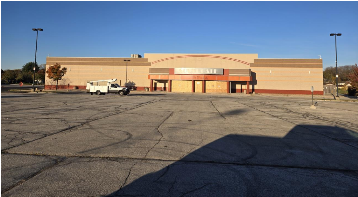
Image 1: East wall of existing building & parking lot
