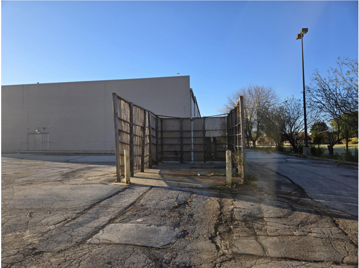
Image 4: Existing dumpster enclosure (to be re-built)
