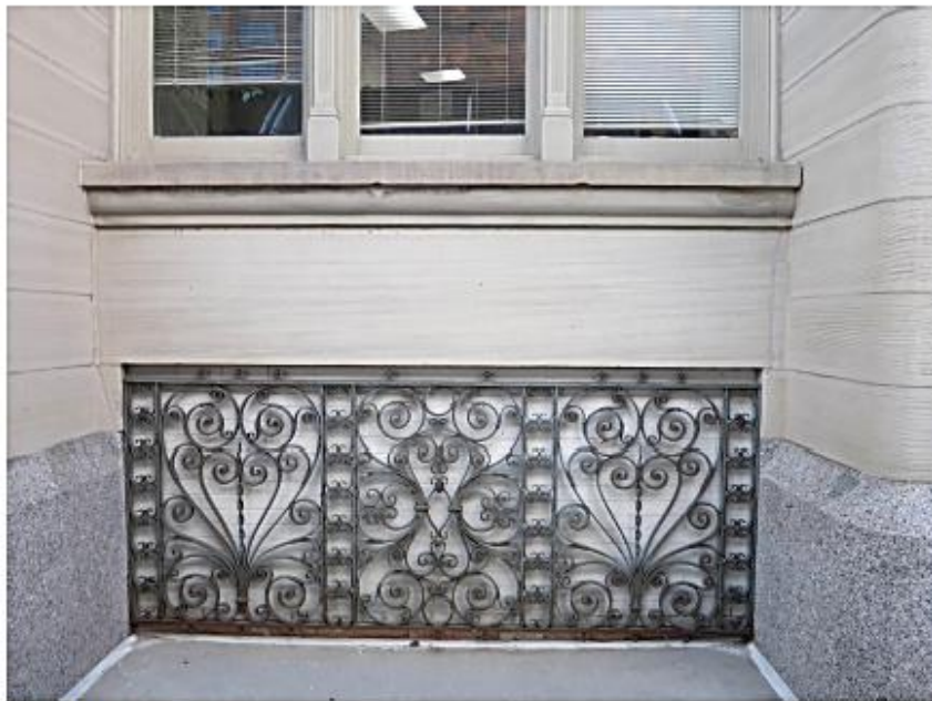
Typical Existing Wrought Iron Grille Work
