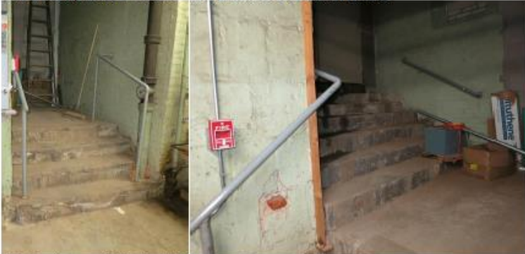
Stair 8 as it enters the Mechanical Room.
