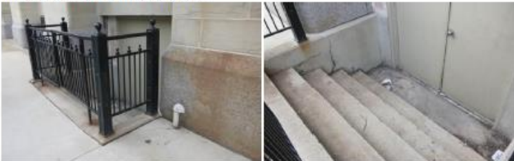
Stair 8 from Market street looking south.
