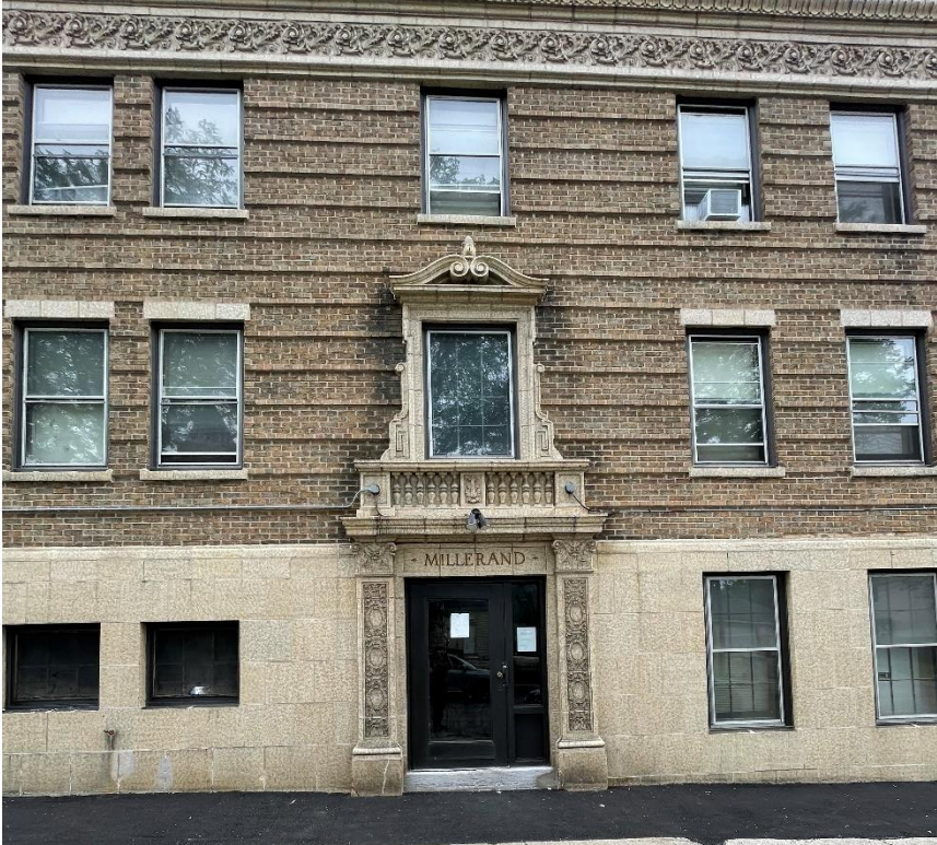
Details of west facade
