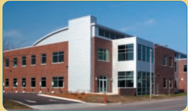
The new Sigma building incorporates a bow truss structure for the main roof, creating open space and a window course for natural light. The selection of building materials complements the neighboring drawbridge and blends with the industrial texture of the Menomonee Valley.
