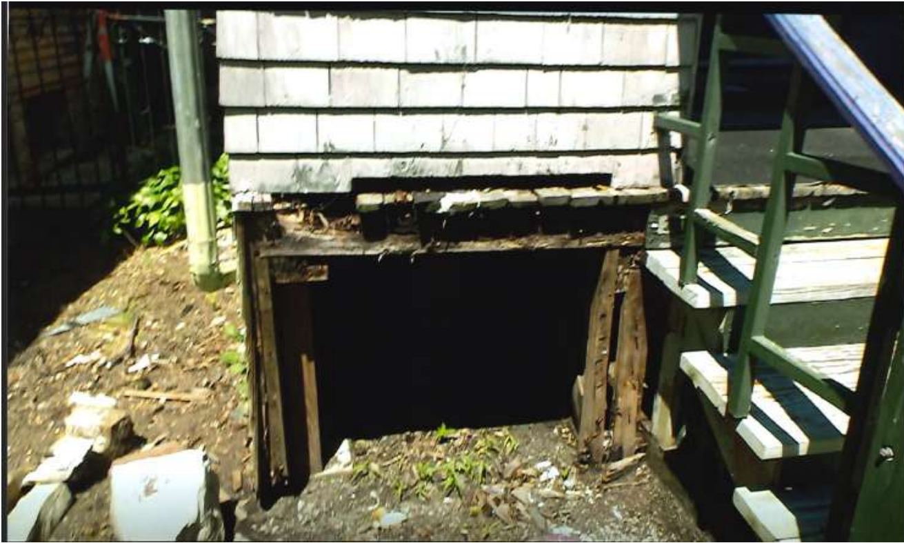
Porch section approved for repair.
