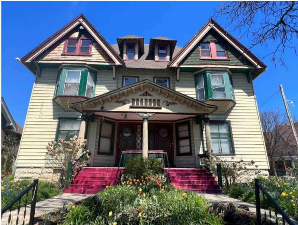
E1 - South Elevation of 2902-04 W State St, facing north
