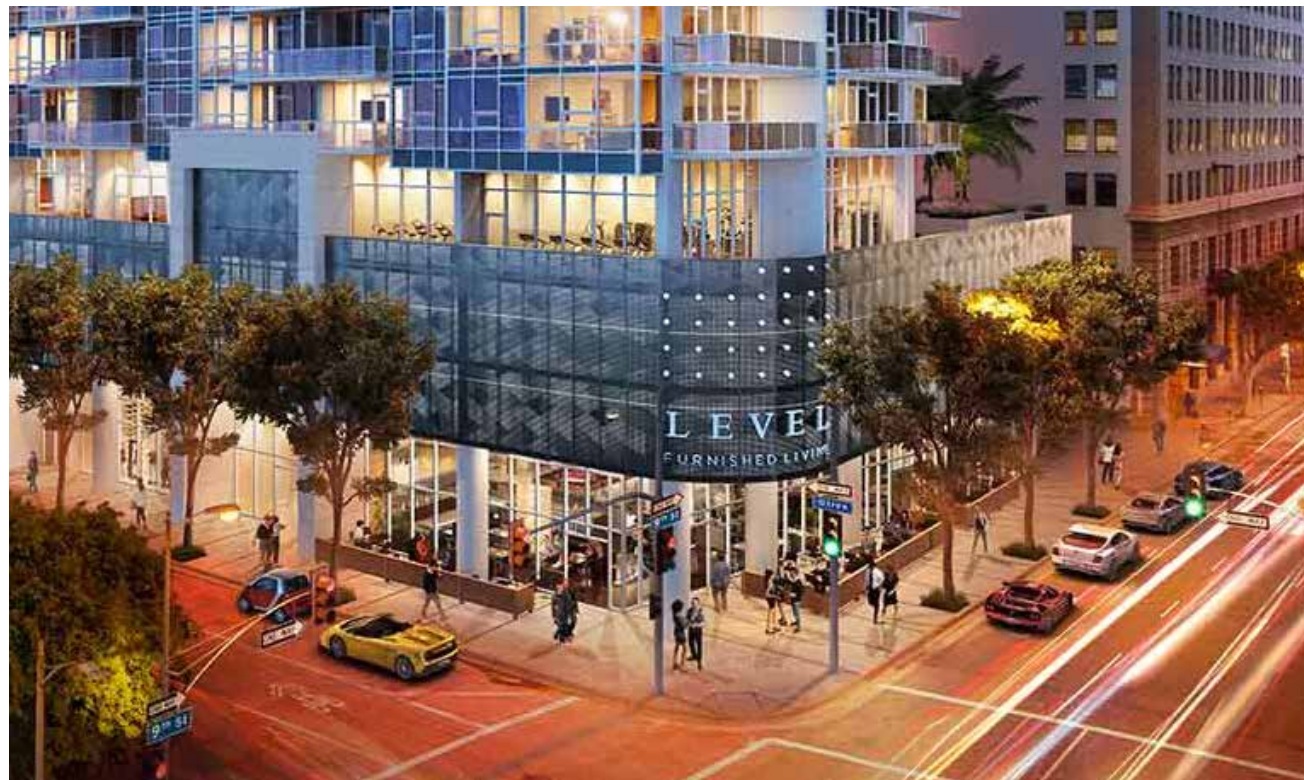
Image 48. Level, Los Angeles (image credit: lamag.com)
