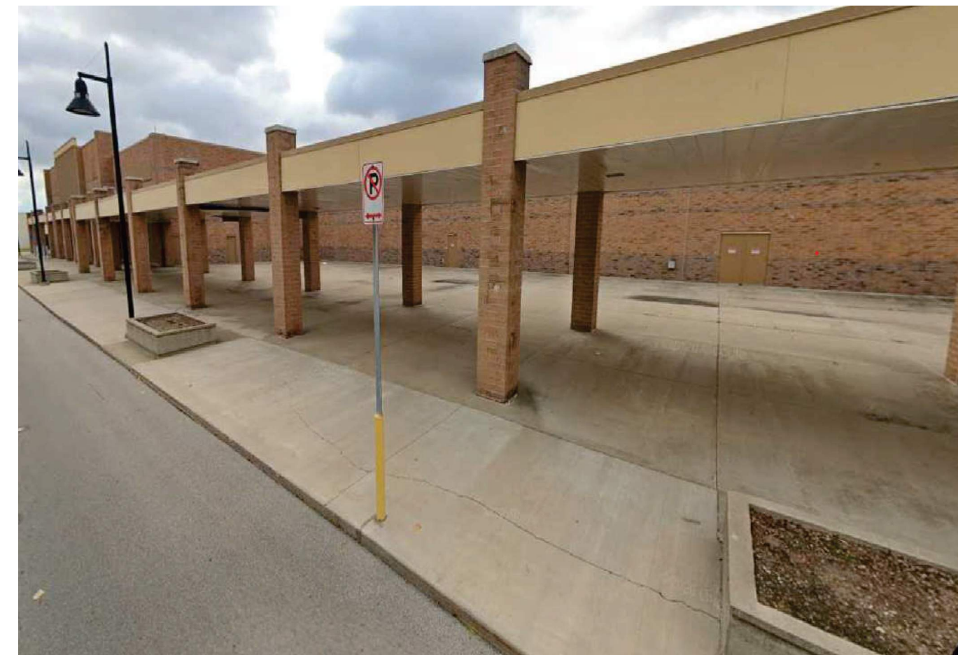
NORTH FACE OF BUILDING - COLONNADE
