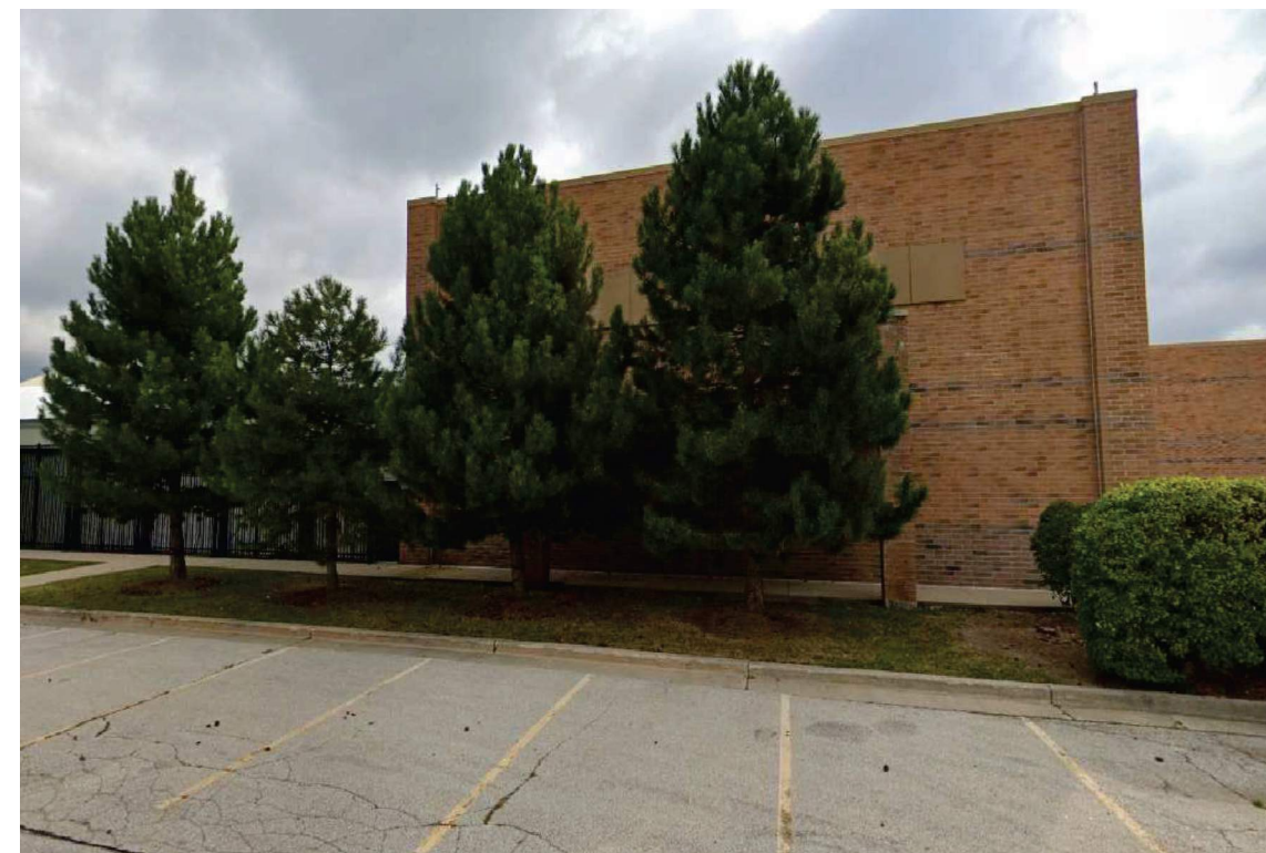
WEST SIDE OF EXISTING BUILDING
