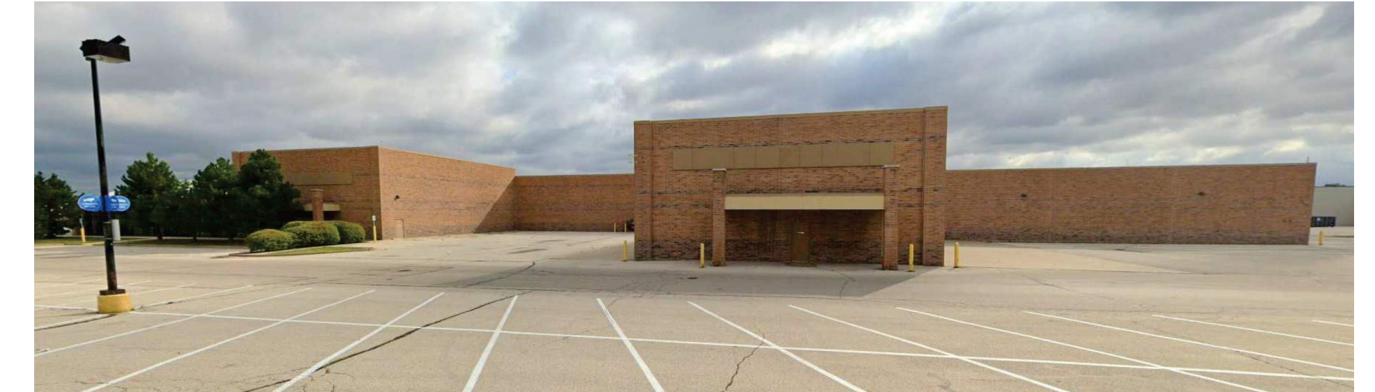
WEST SIDE OF EXISTING BUILDING
