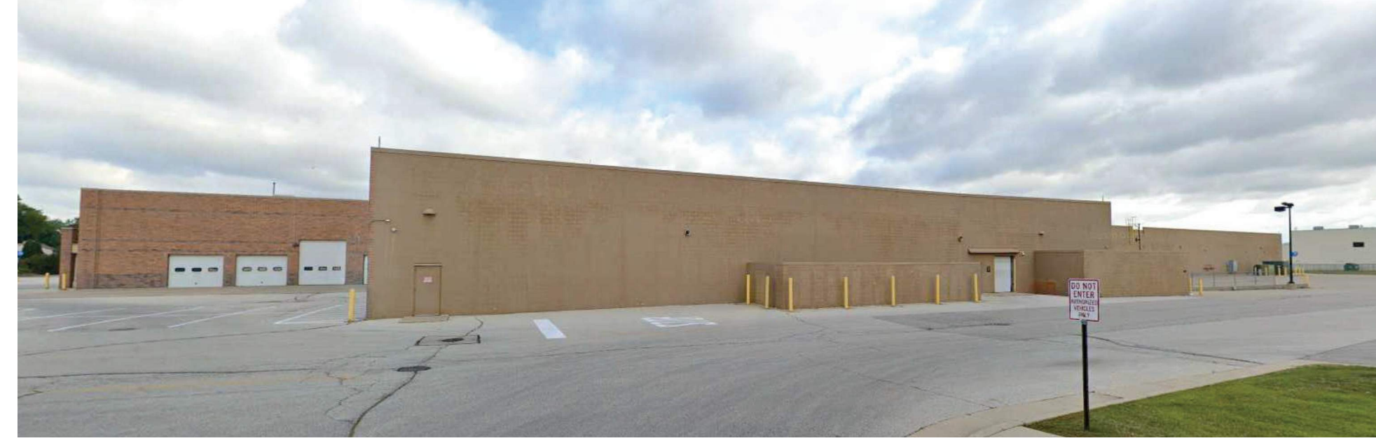
SOUTH SIDE OF EXISTING BUILDING
