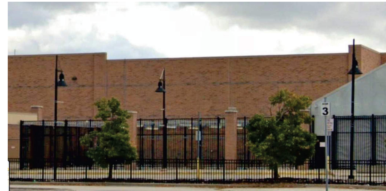
NORTH SIDE OF EXISTING BUILDING - WEST END
