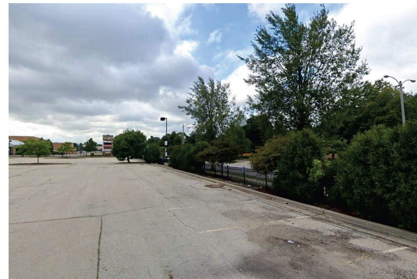
LOCATED AT NORTHWEST CORNER OF NORTH PARKING LOT LOOKING SOUTH ALONG N 60TH ST.
