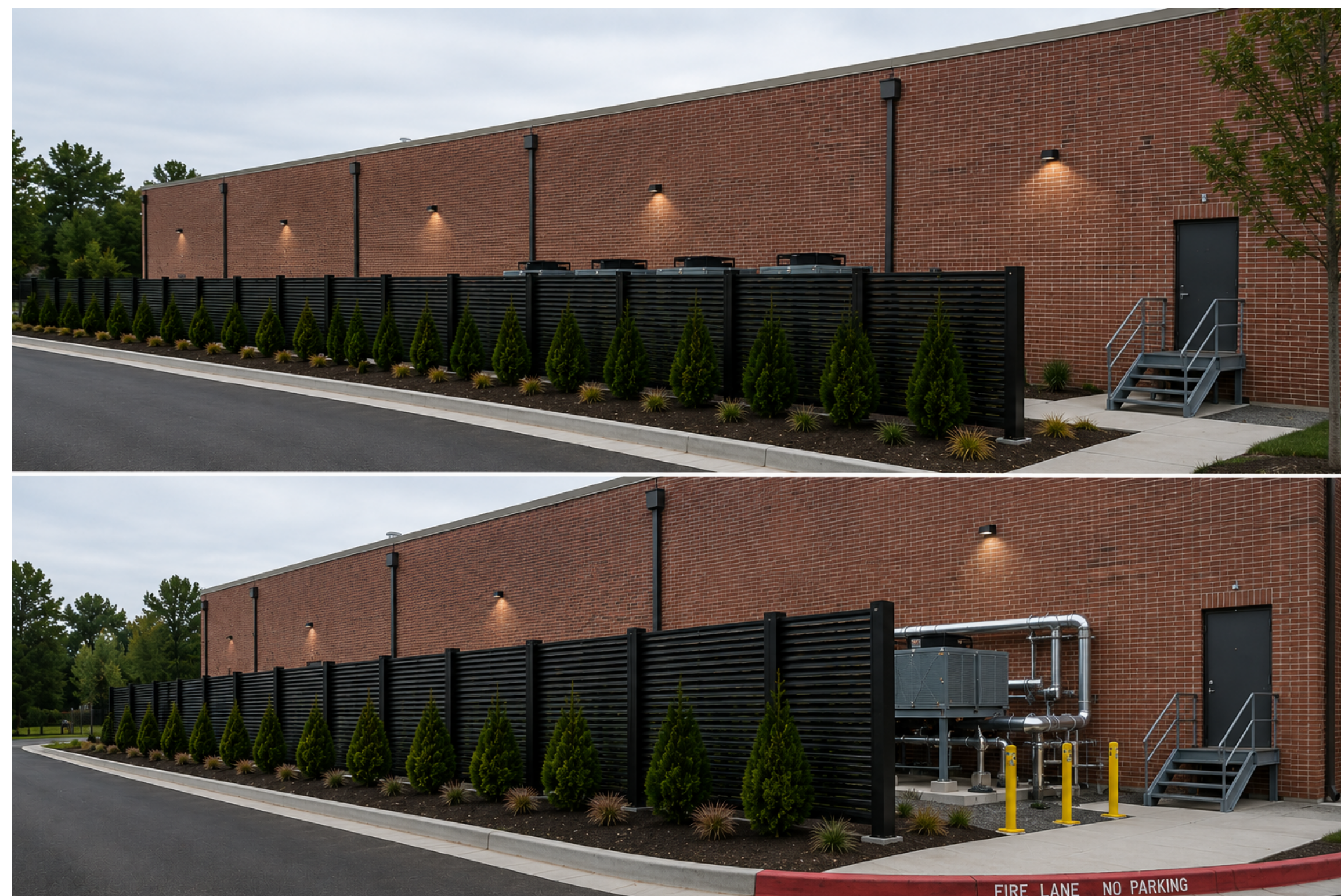
EXAMPLE OF ENGINEERED ACOUSTIC SCREENING WALL SYSTEM
