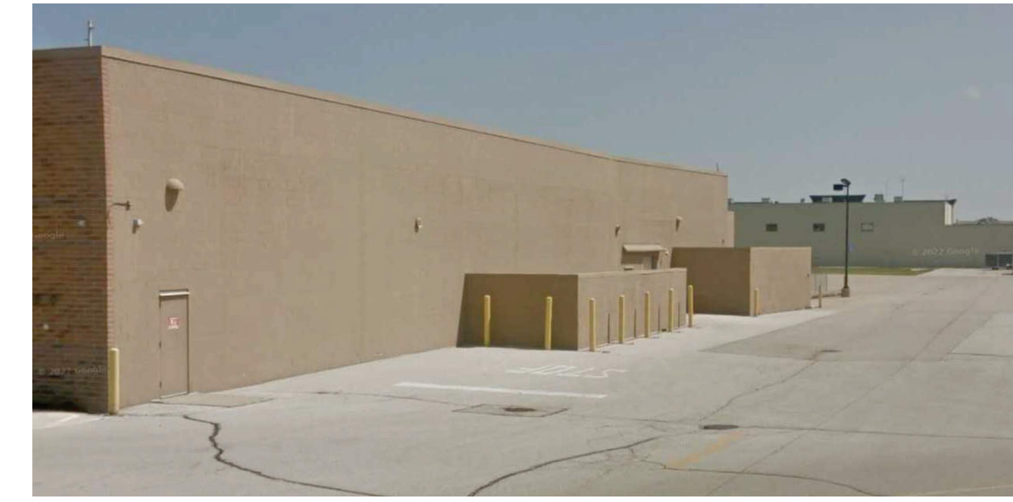
SOUTH SIDE OF EXISTING BUILDING
