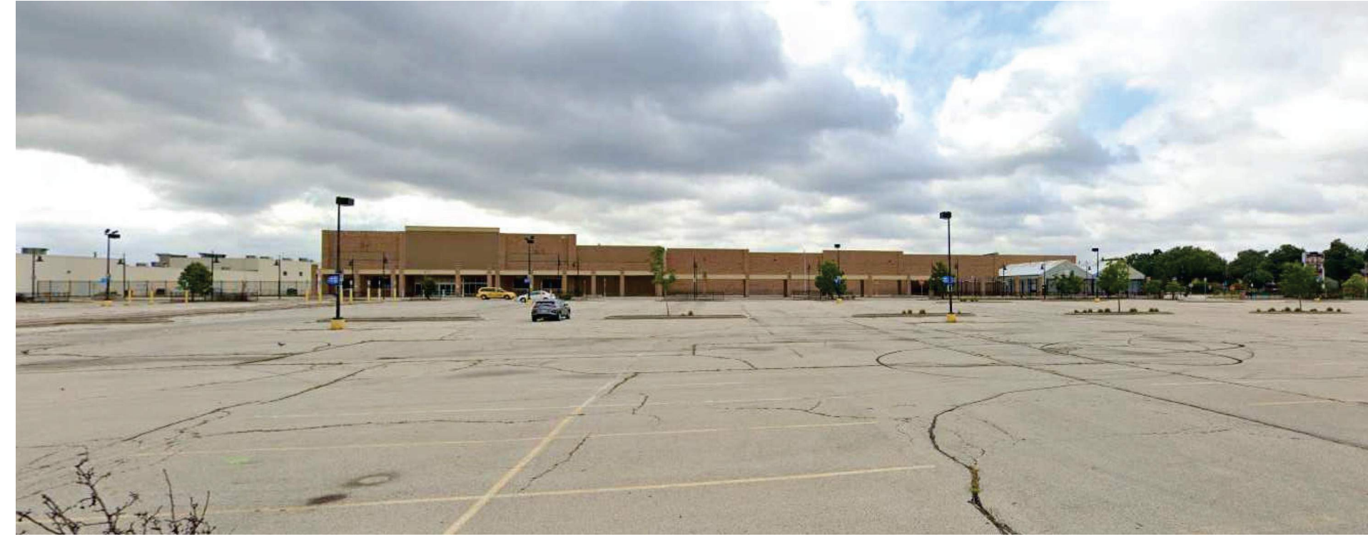
NORTH FACE OF EXISTING BUILDING
