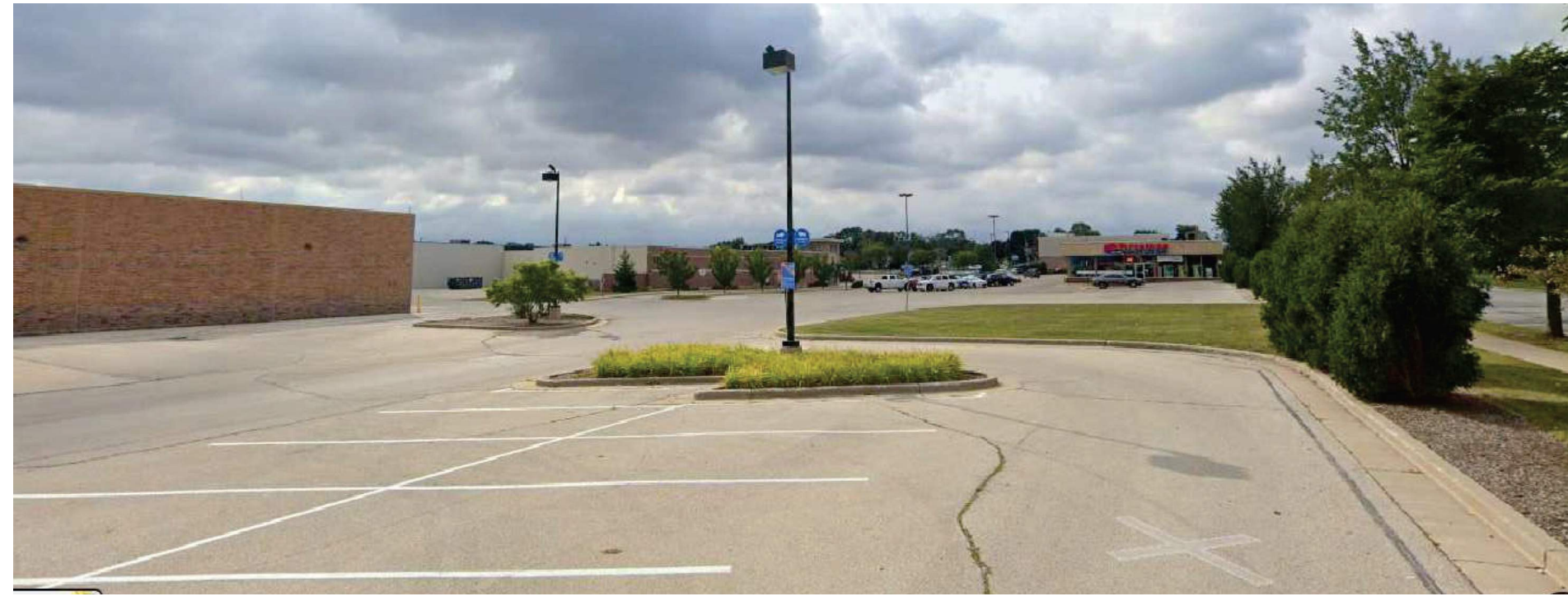
SOUTHWEST CORNER OF EXISTING BUILDING
