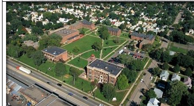
Aerial view of the St. Paul Minnesota Center
