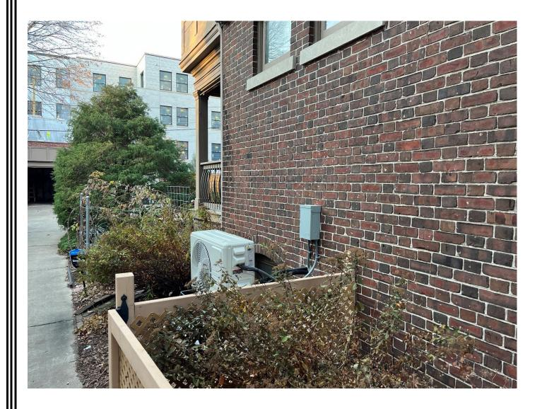
Location of mini split heat pump connection, screened from view by existing fence.
