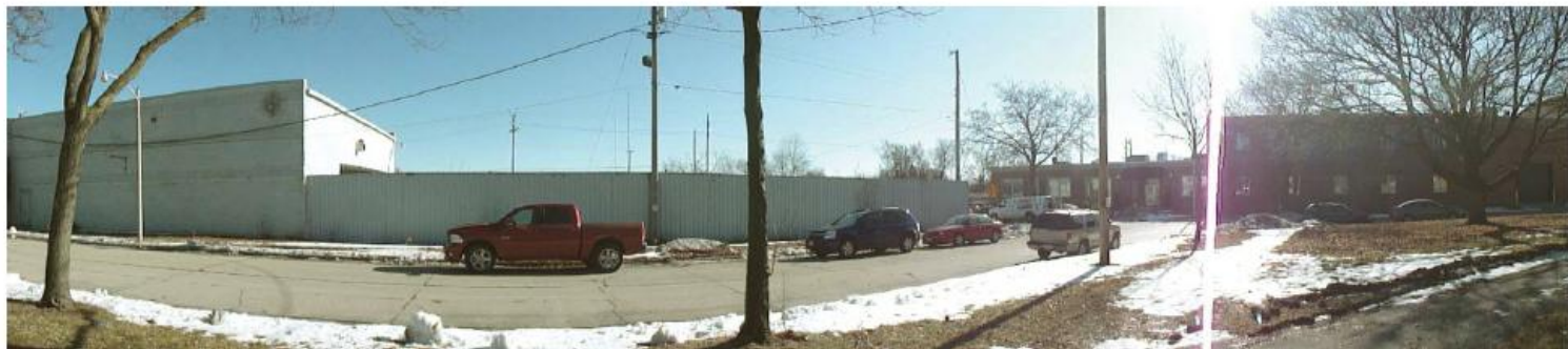
View: West edge of acquired property and view of the north facade of the existing Novozymes facility.
