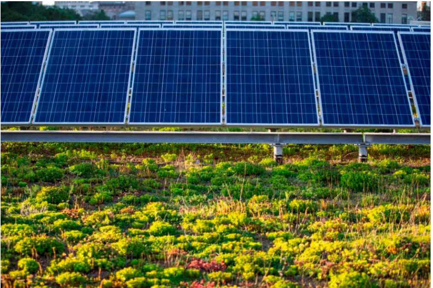
Milwaukee Public Library's Green Roof.
