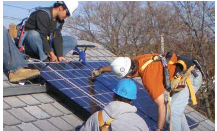
Rooftop solar installation. Photo Credit: MREA
