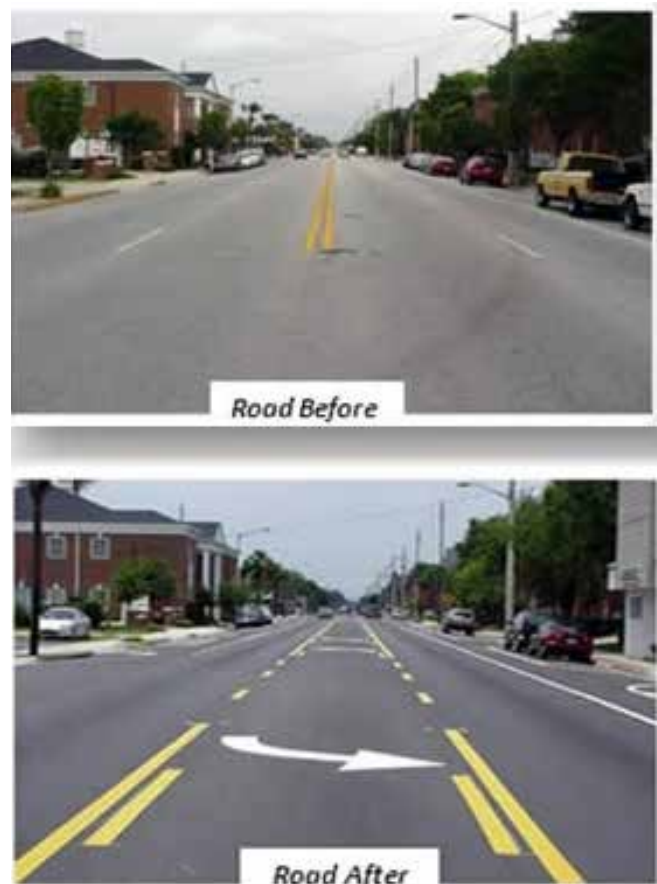
Example of possible design changes to prioritize safer walking. Image by the Federal Highway Administration.
