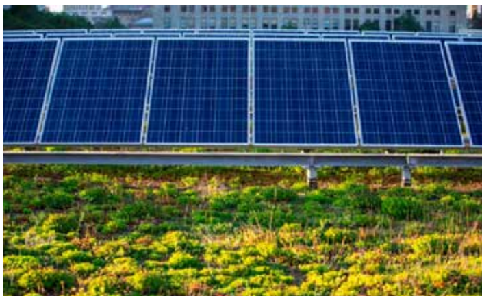
Solar panels on top of Milwaukee Central Library.
