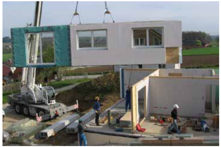
Modular housing being transported to the build site.
