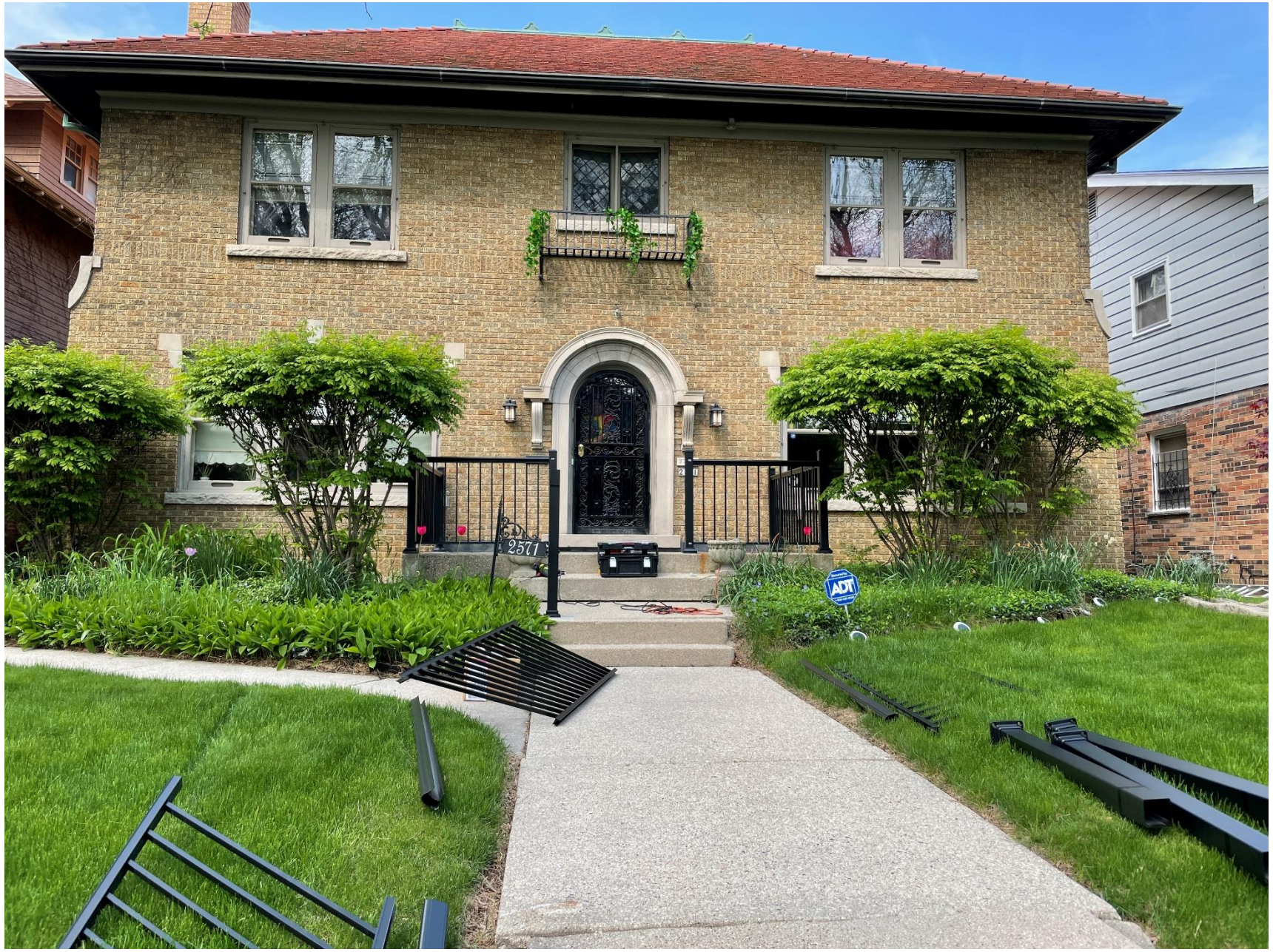
New railings under construction.
