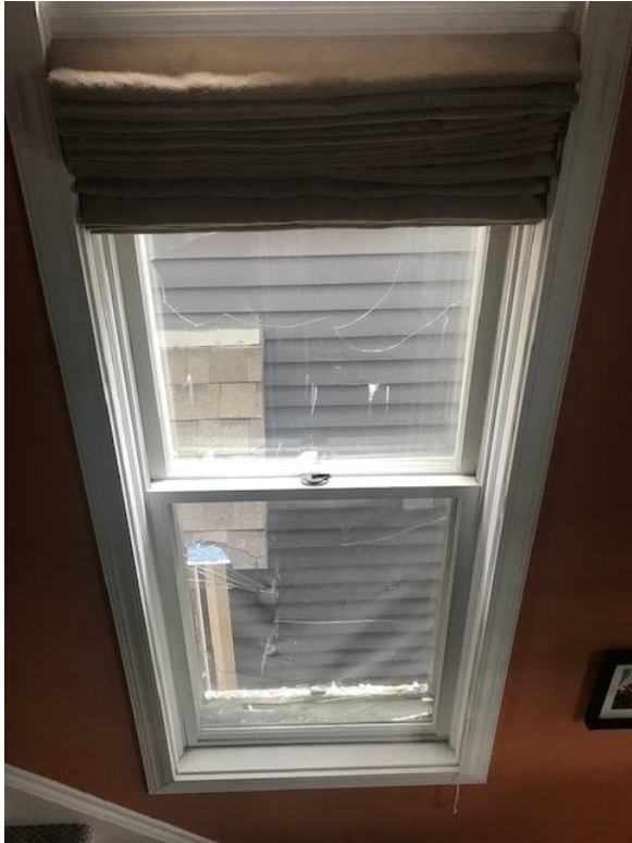
NE Side Window – Interior
