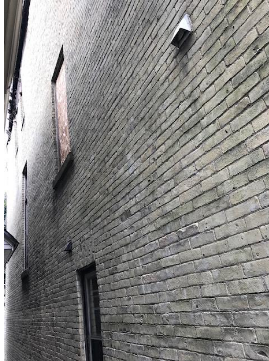
NW Window - Exterior
