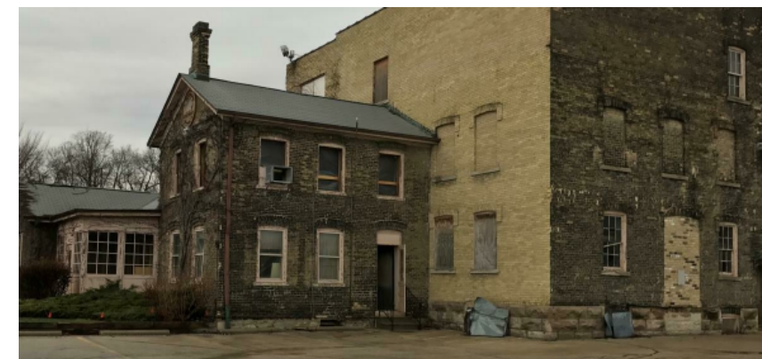
9 CURRENT CONDITIONS (PHOTO FROM THE REVISED HISTORIC DESIGNATION STUDY REPORT) 1 1/2" = 1'-0"
