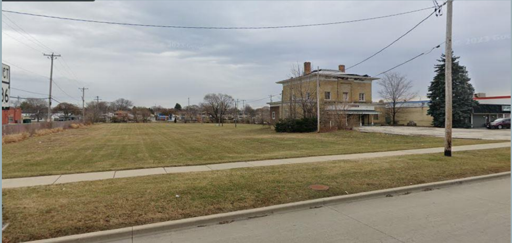
Existing building as viewed from South 27 th Street
