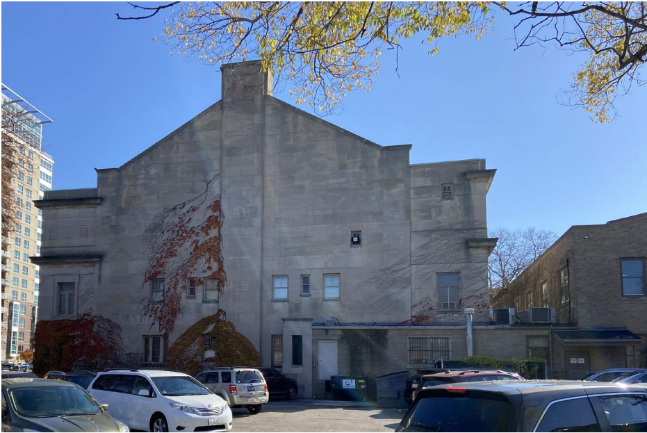
Existing 1451 N Prospect (Renaissance Place) - West Facade
