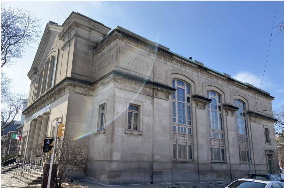
Existing 1451 N Prospect (Renaissance Place) - North Facade
