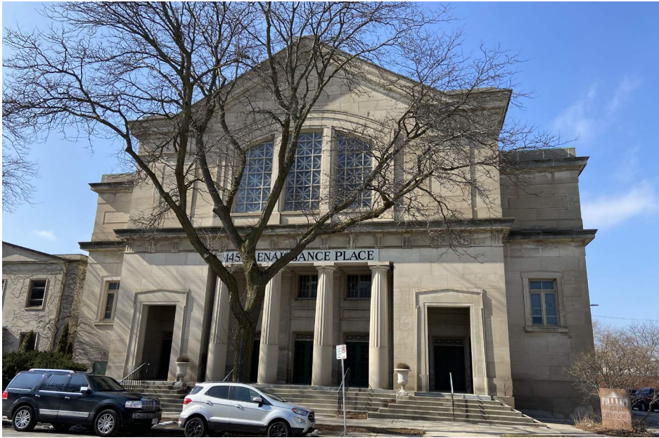
Existing 1451 N Prospect (Renaissance Place) - East Facade & Building Signage
