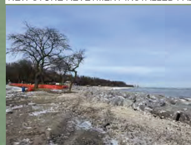
NEW STONE REVETMENT INSTALLED FALL 2024
