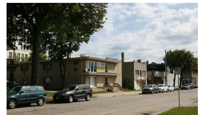
SOUTH EAST CORNER
