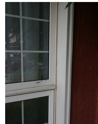
FRONT REPLACED WINDOW
