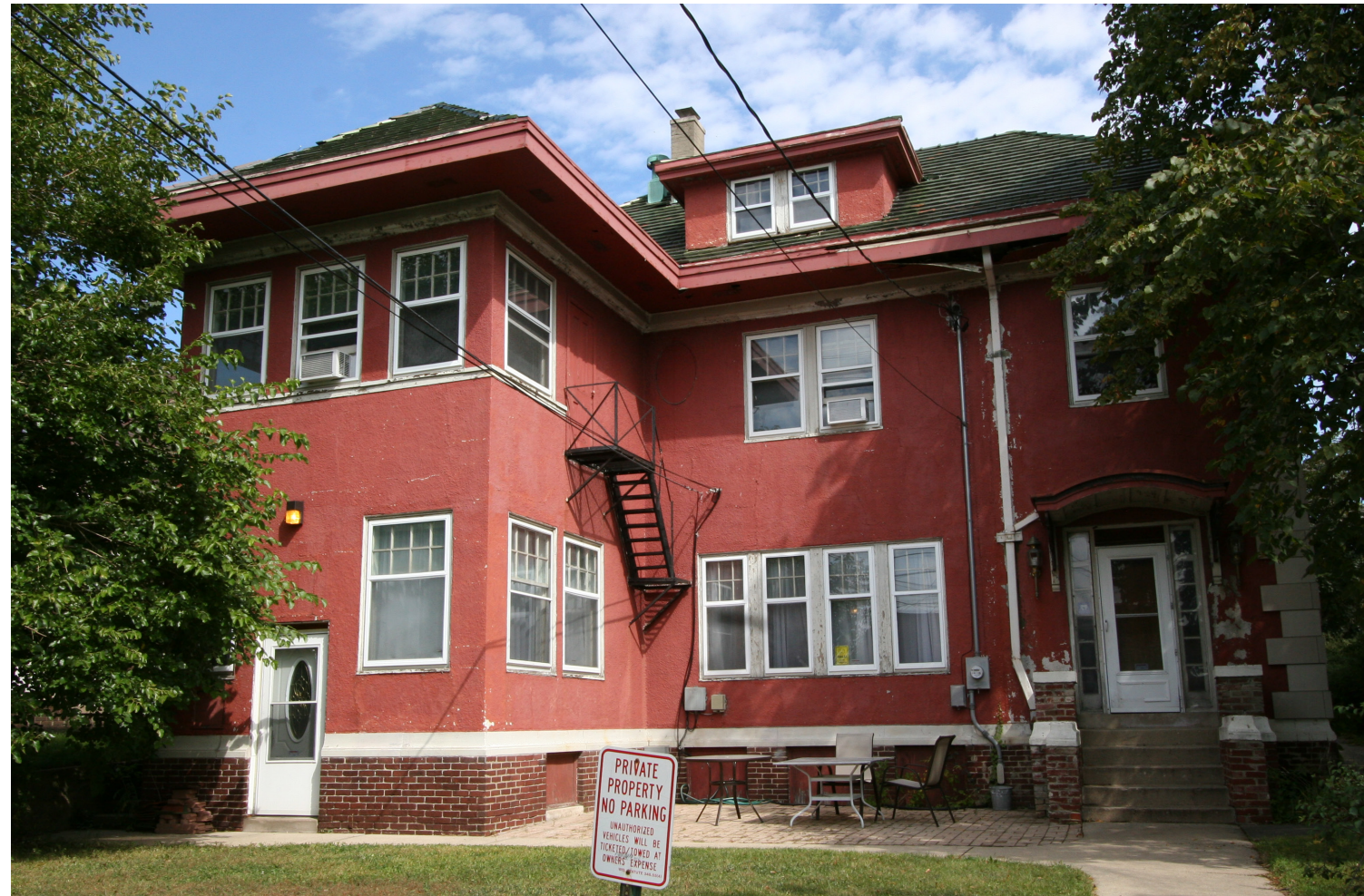
REAR (ALLEY) ELEVATION LOOKING EAST
