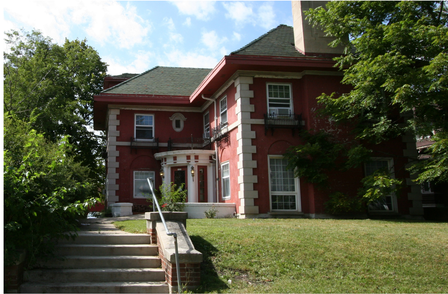
STREET ELEVATION LOOKING WEST
