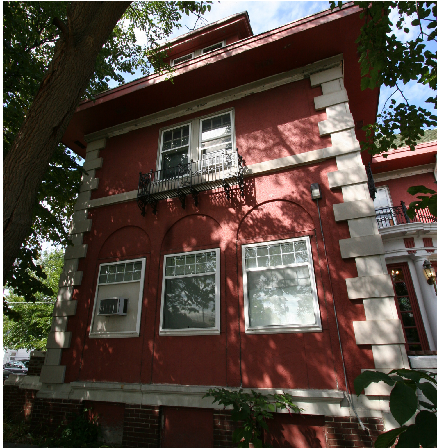
SOUTH SIDEYARD ELEVATION LOOKING NORTH
