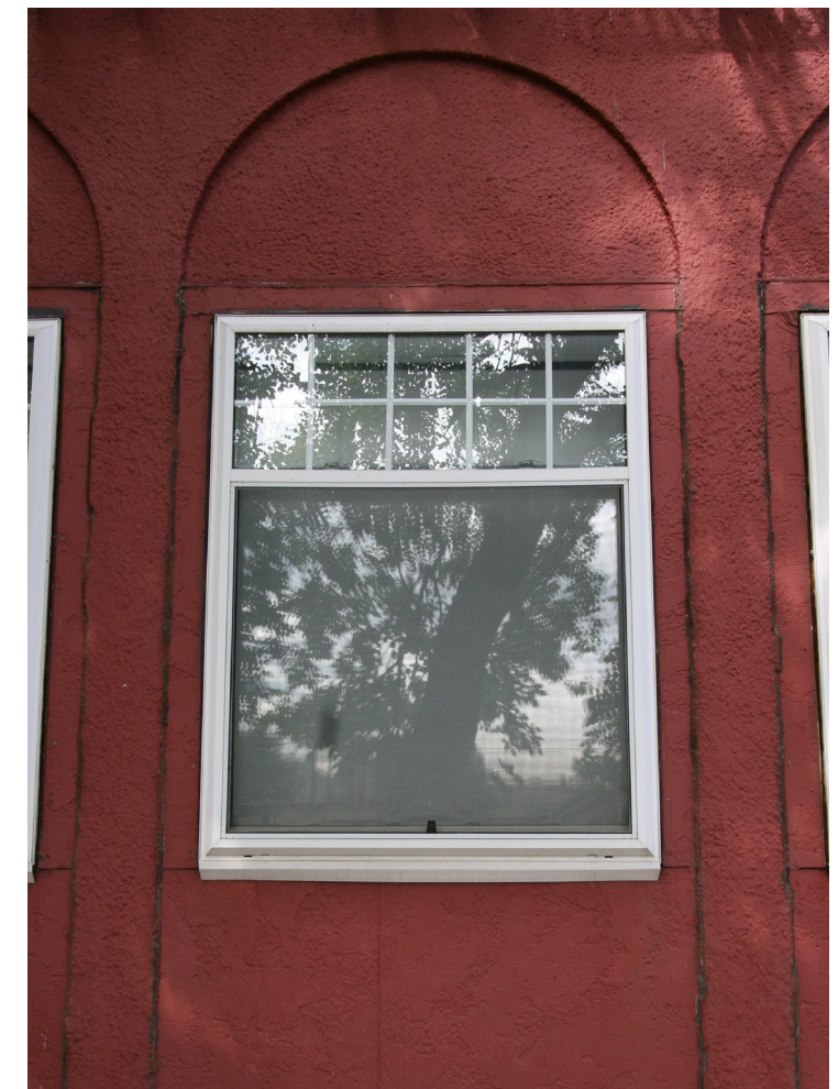
SOUTH FIRST FLOOR WINDOW DETAIL
