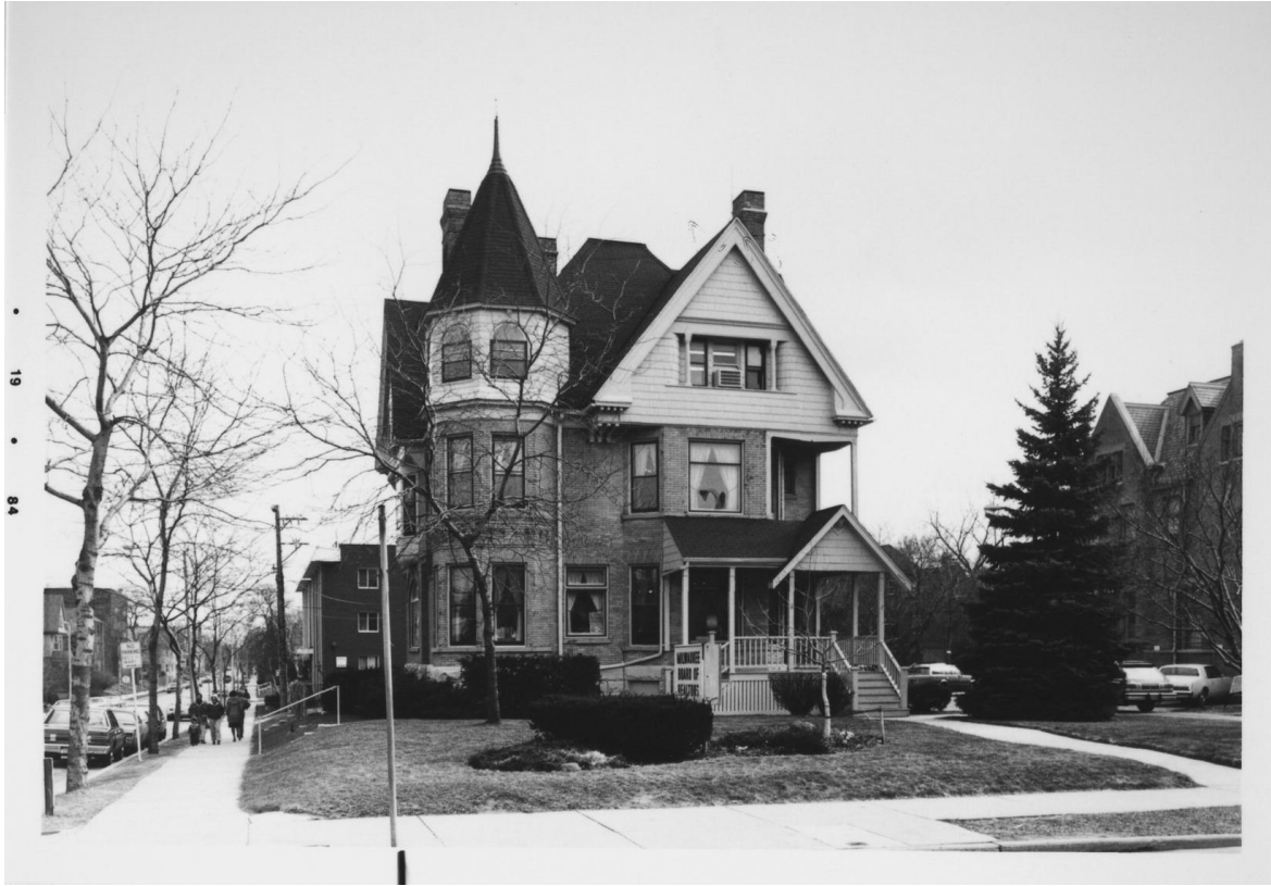
Wisconsin Architecture and History Inventory, Record #42026. Photo taken 1984.
