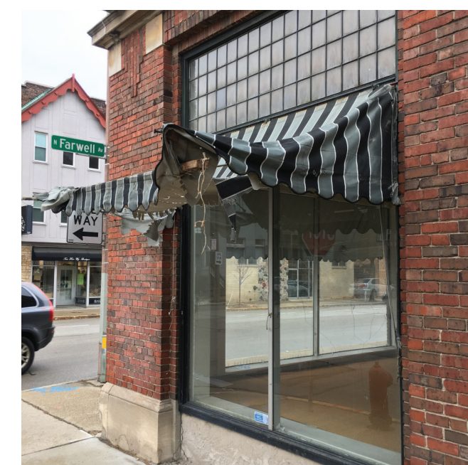
EXISTING FABRIC AWNING
