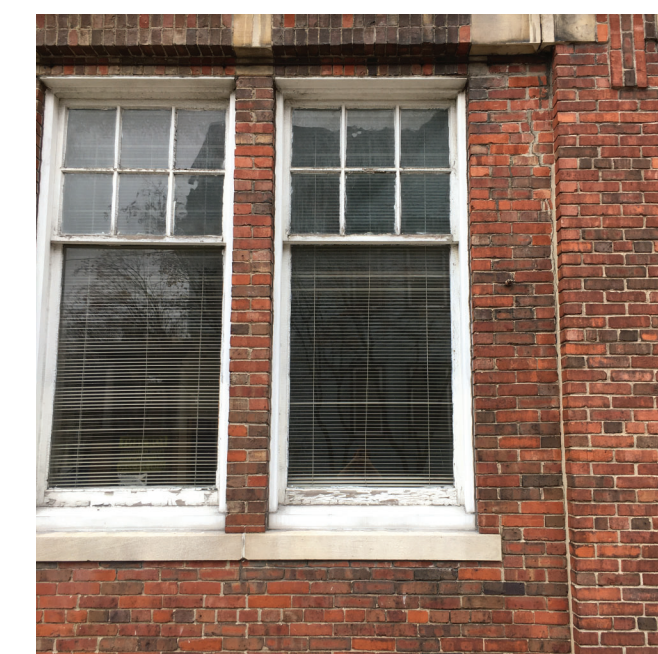
EXISTING MASONRY & WINDOWS
