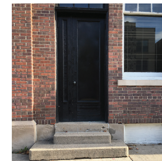
EXISTING DOORS & WINDOWS
