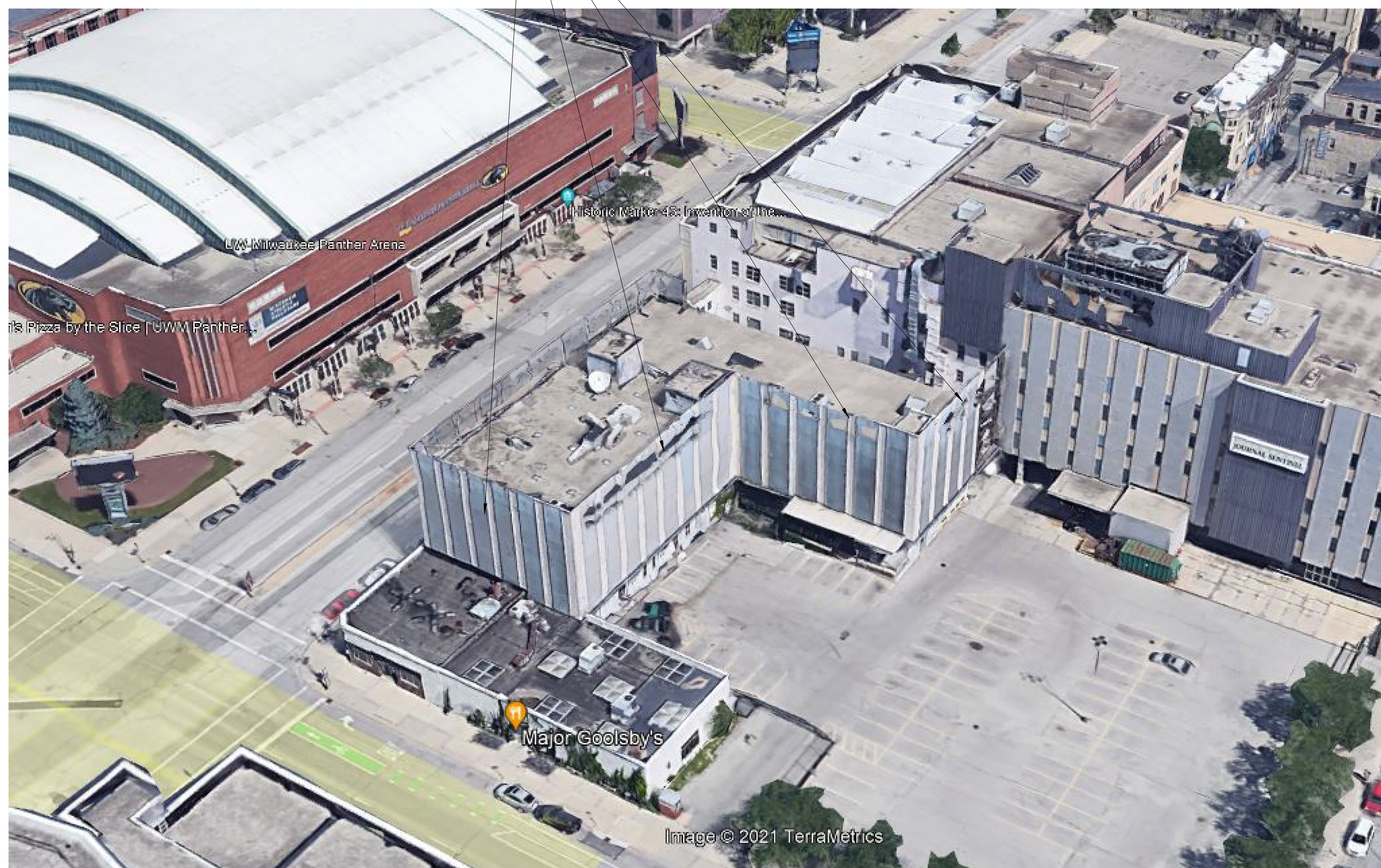
CURRENT SOUTH AERIAL
