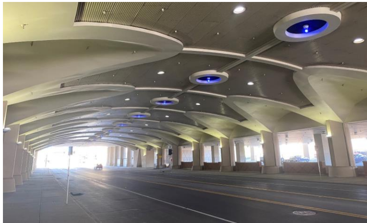
EXISTING CONDITIONS LOOKING WEST
