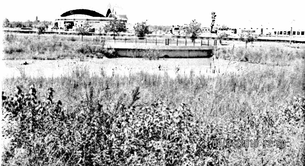
Bio-Retention Facility at 35 th and Canal
