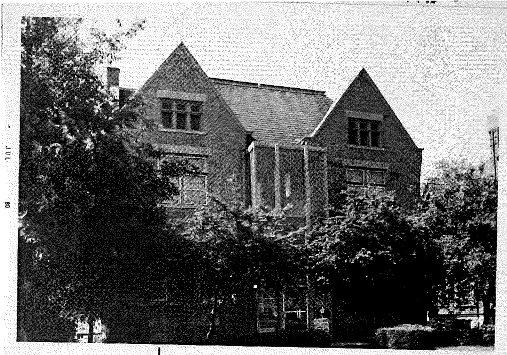
Wisconsin Architecture and History Inventory, Record #42027. Photo taken 1980.
