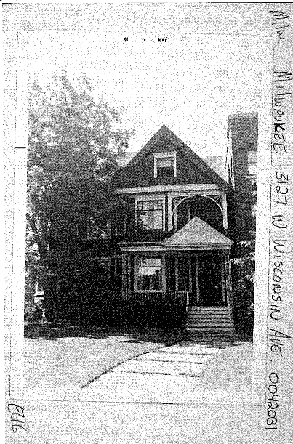
Wisconsin Architecture and History Inventory, Record #42031. Photo taken 1980.
