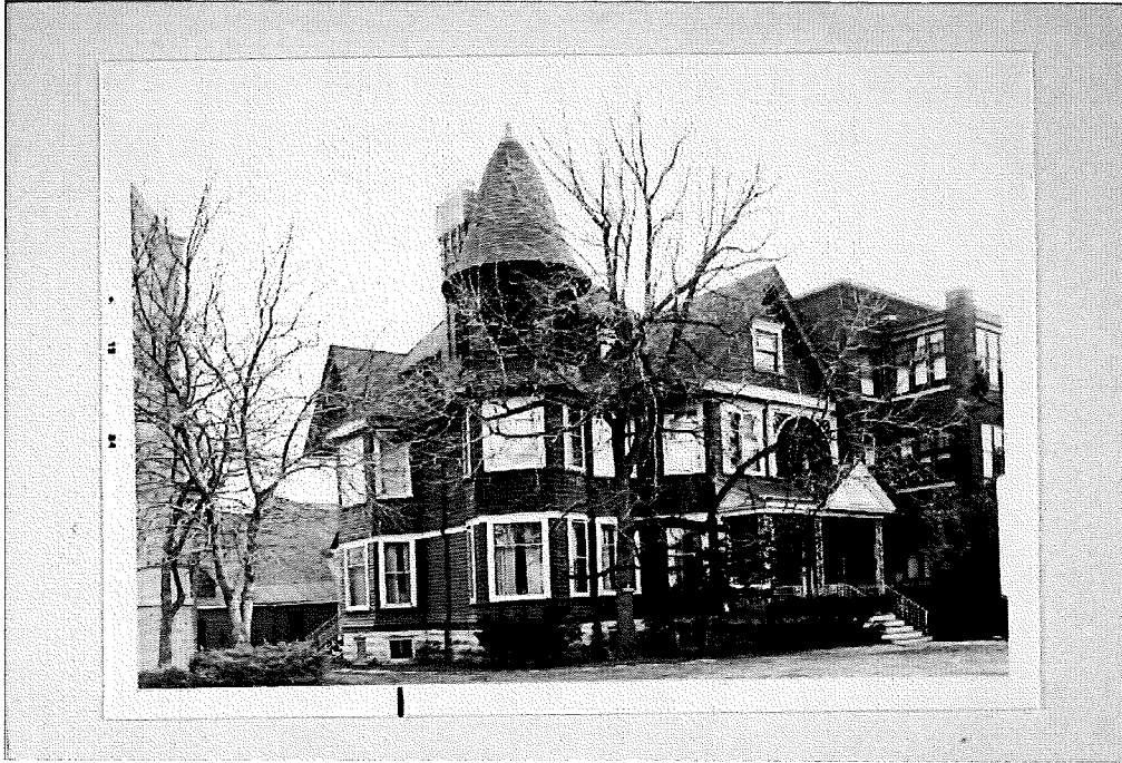
Wisconsin Architecture and History Inventory, Record #42031. Photo taken 1984.
