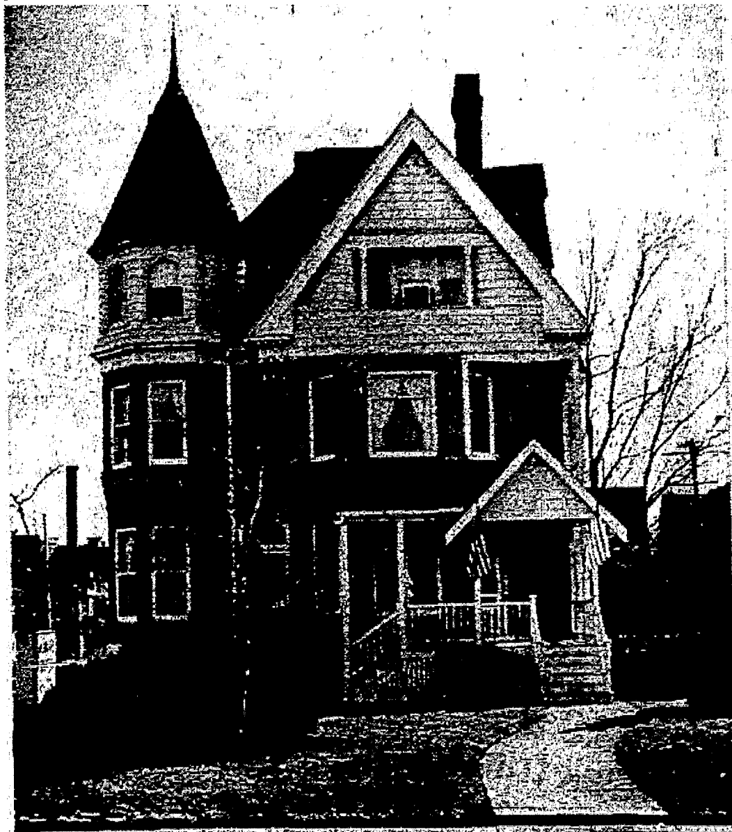
The exterior of the Realtors' building, a home built in 1892, has been restored to its turn of the century appearance. The original porch was duplicated; asphalt siding was replaced by cedar shake shingles on the third floor, the Cream City brick was cleaned and a new roof was added. —Journal Photo
