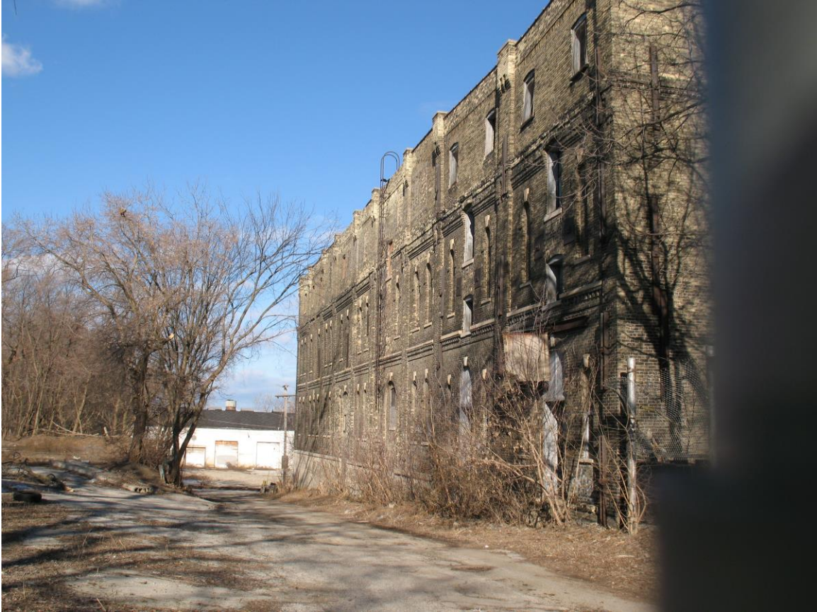
South Elevation Ice House/Malt House
