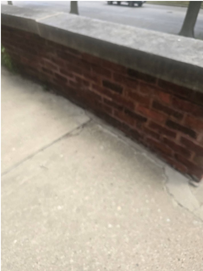
Brick to be tuck pointed, where needed
