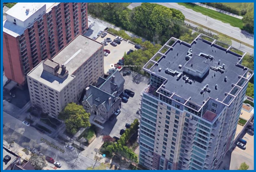
Tilt view from North Prospect Avenue, looking northeast
