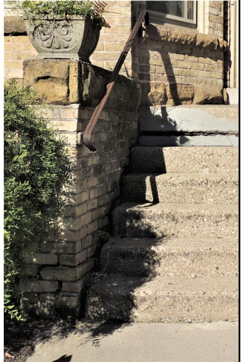
Stair condition detail. Note deterioration at left/south
