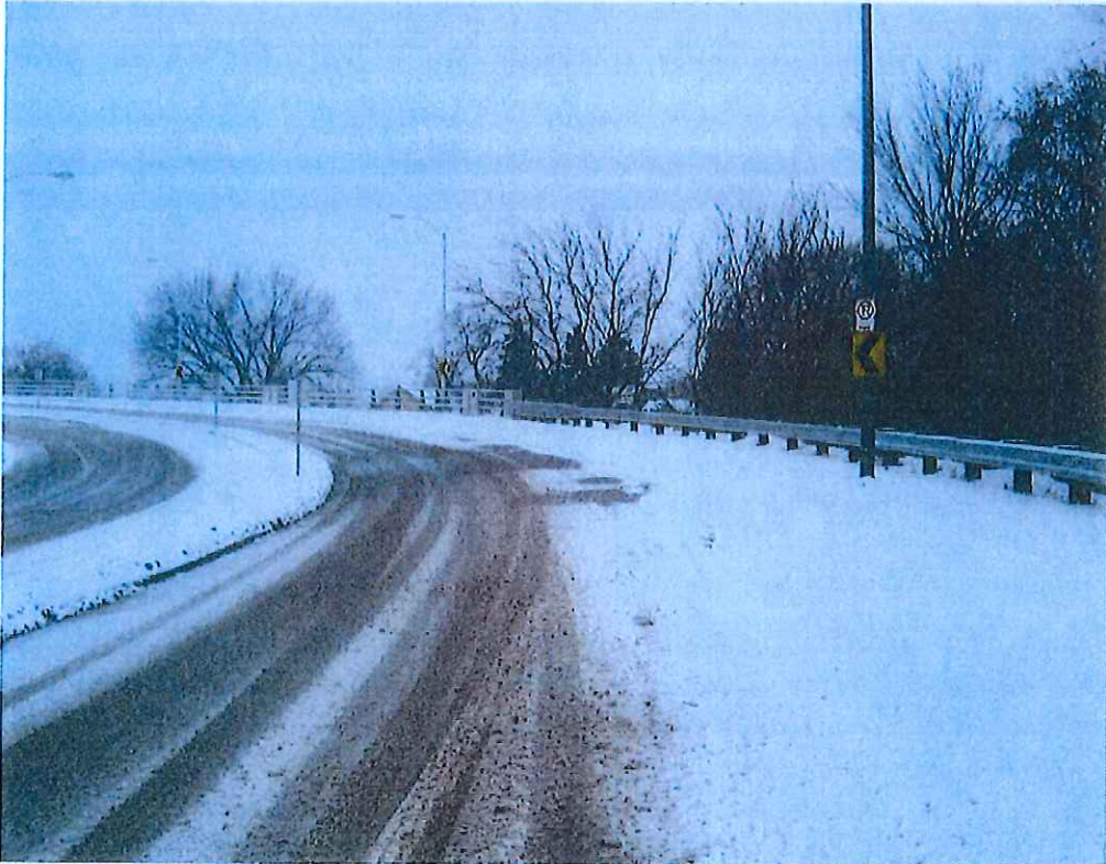
2100 S Bay St - bridge Eastbound 12-14-13 1107 hr.jpg
