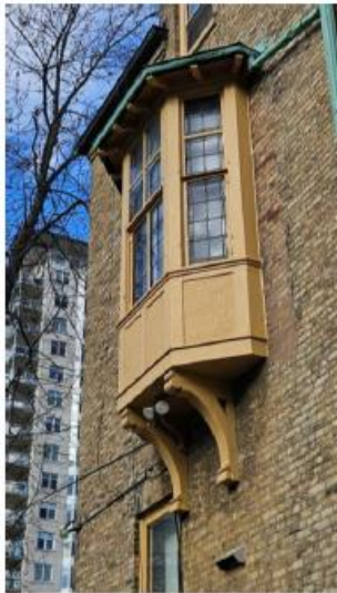
Bracket Detail And Existing Dormer Gable
