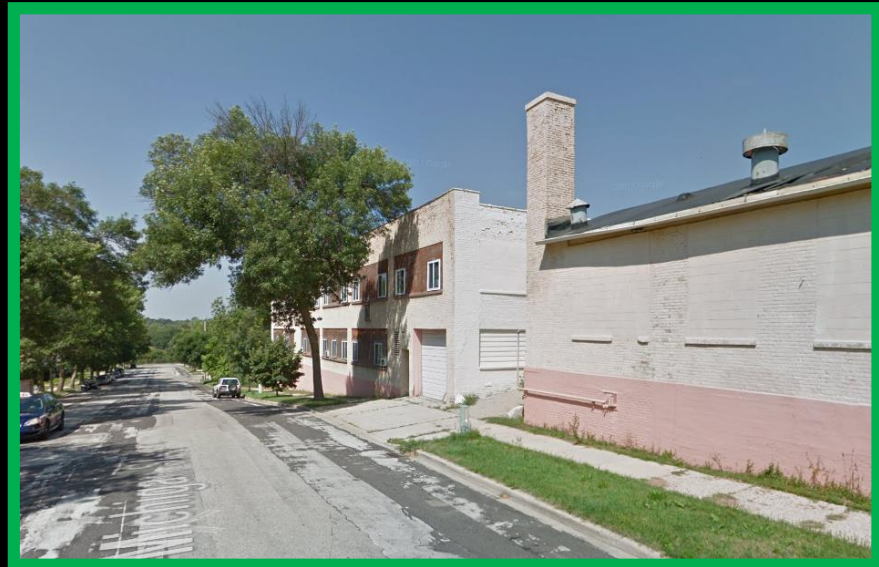
View from West Michigan looking east
