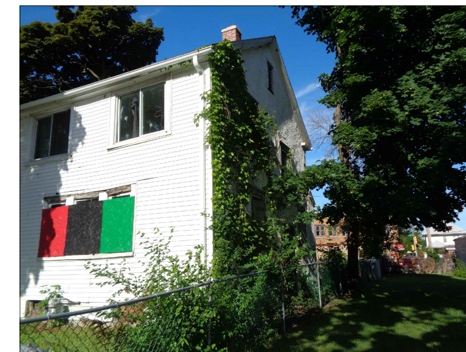
EXISTING NORTHEAST CORNER
