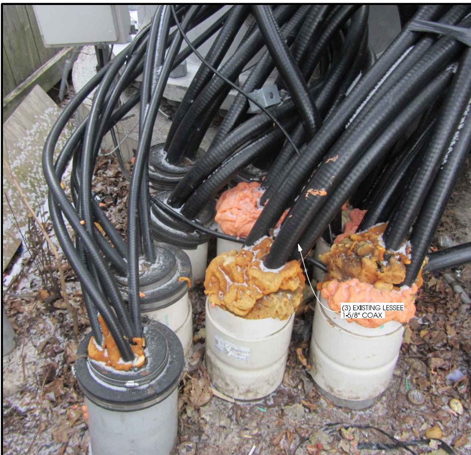
COAX PORT LAYOUT (SHELTER EXTERIOR)
