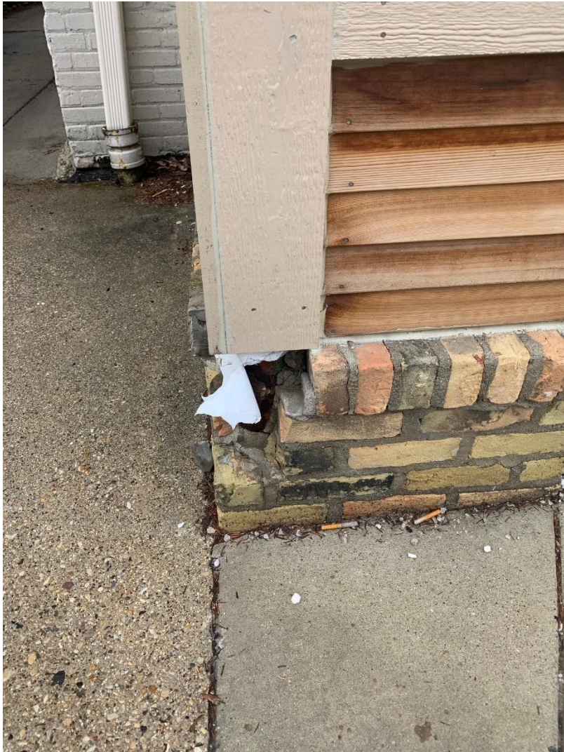
Areas to be repointed and repaired
