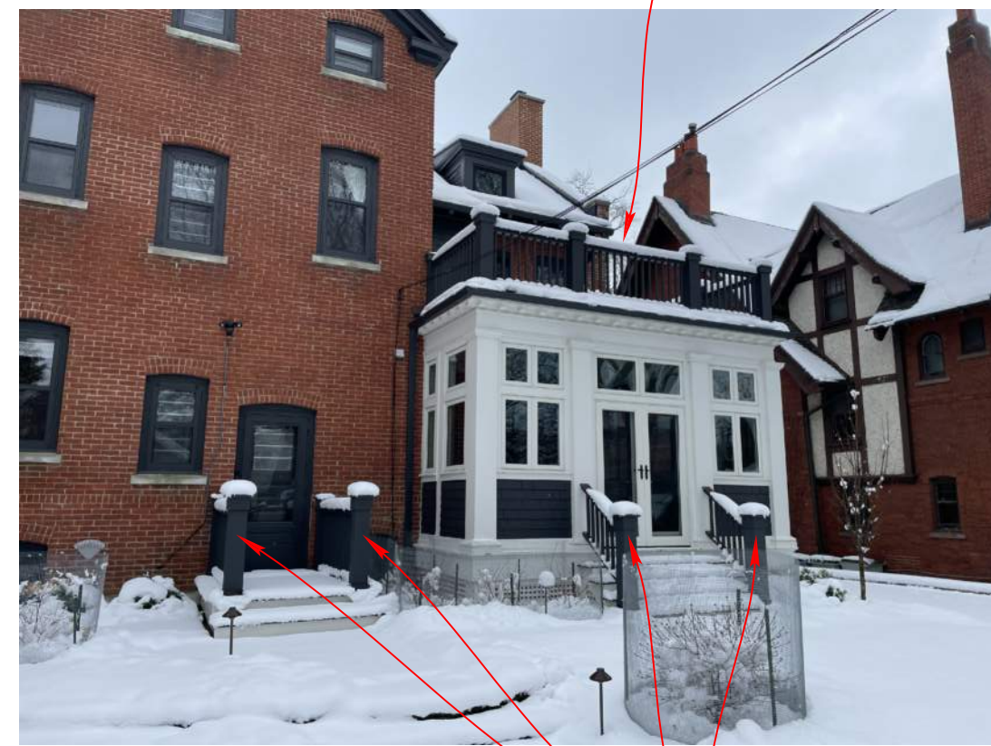
PHOTO 2 REAR PORCH AS SEEN FROM BACK YARD
