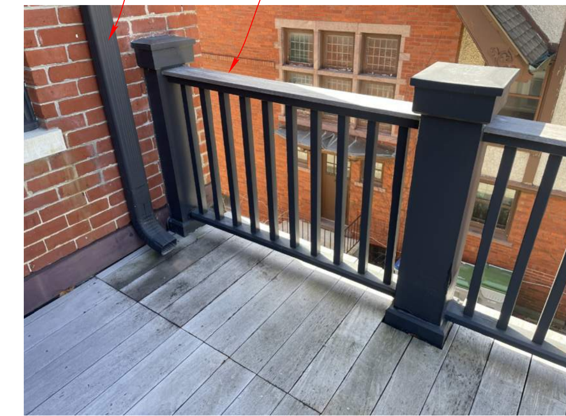
PHOTO 5 ROOF DECK AT MAIN HOUSE
