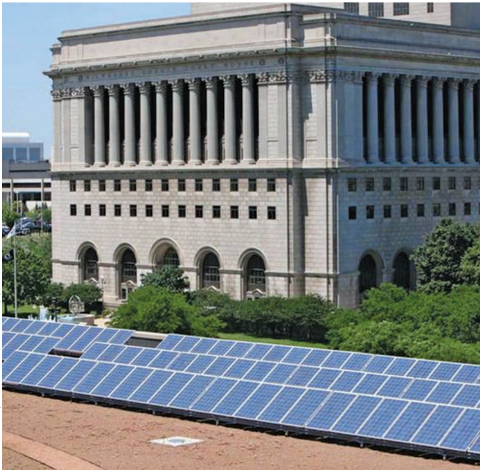
Milwaukee Central Library solar installation. Photo: Donald M. Murphy
