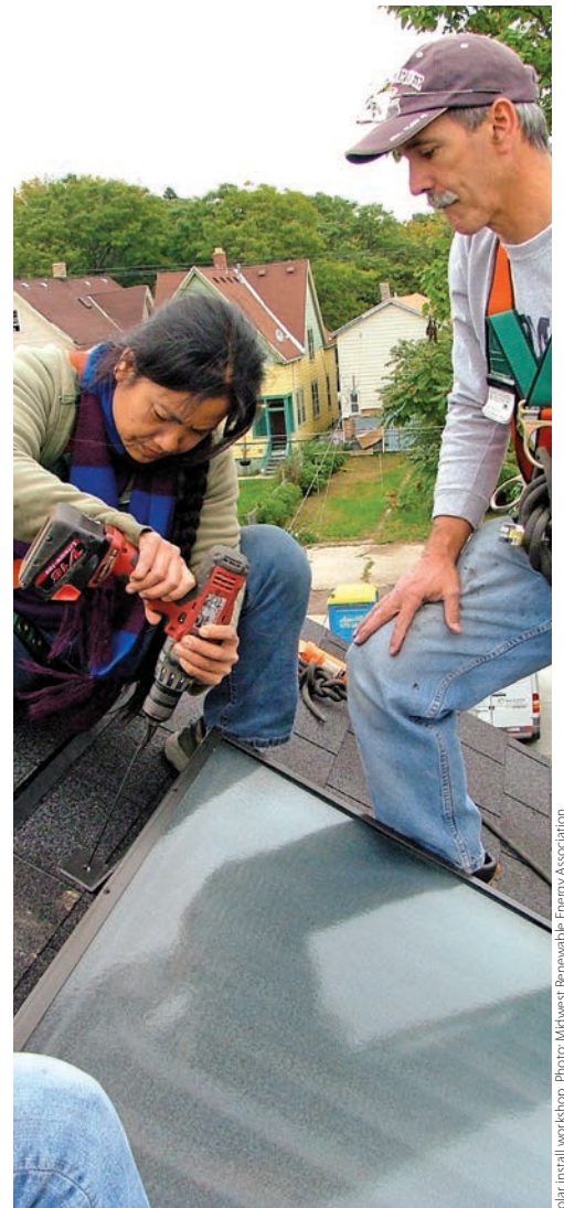
Solar install workshop. Photo: Midwest Renewable Energy Association
