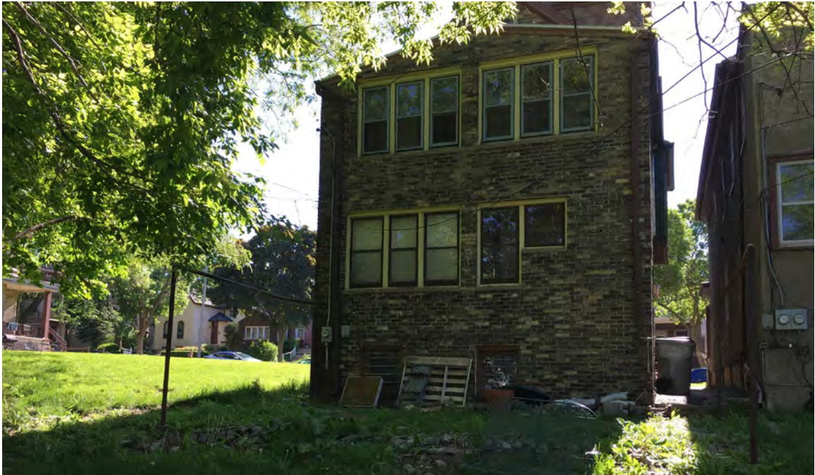
13. VIEW OF PROJECT SITE - LOOKING EAST FROM ALLEY
