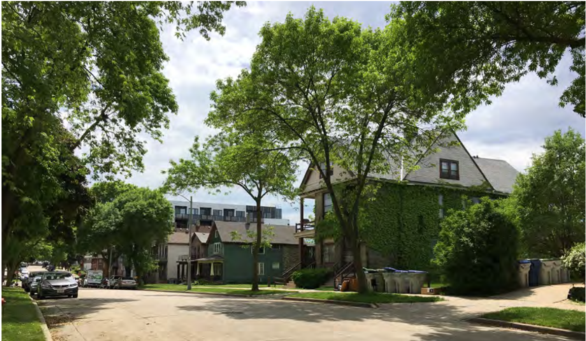
11. VIEW OF PROJECT SITE - LOOKING SOUTHWEST FROM JACKSON ST
