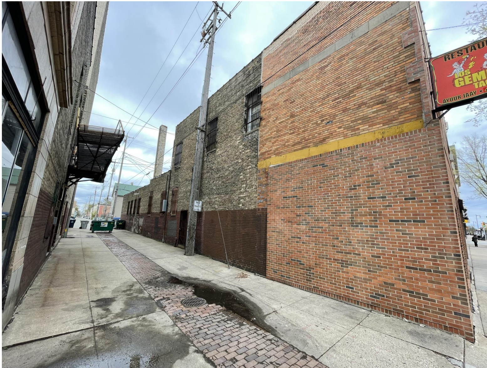
Installation site at right.
