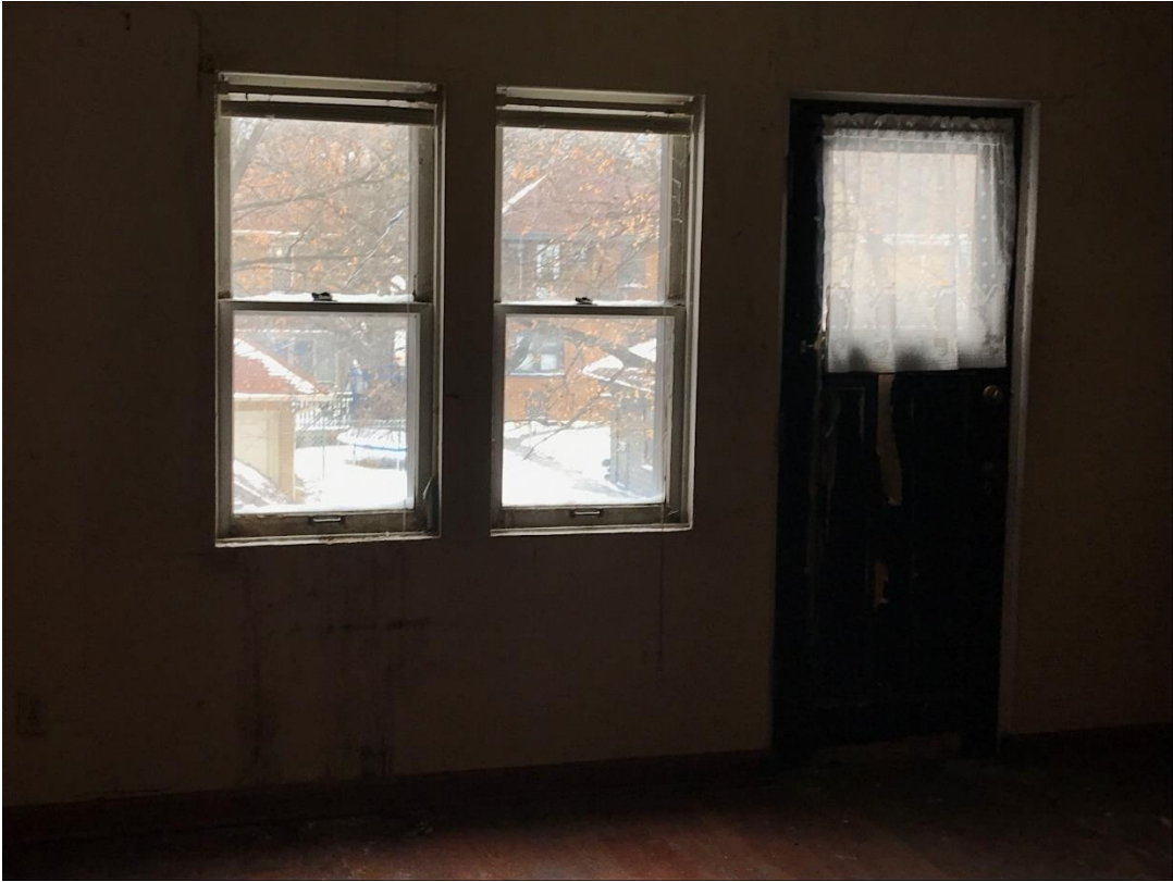
Upstairs Back Windows:
