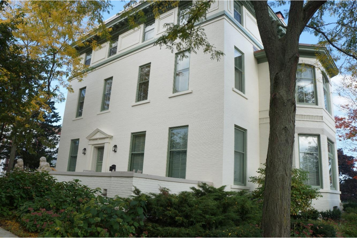
South Elevation, West Portion
