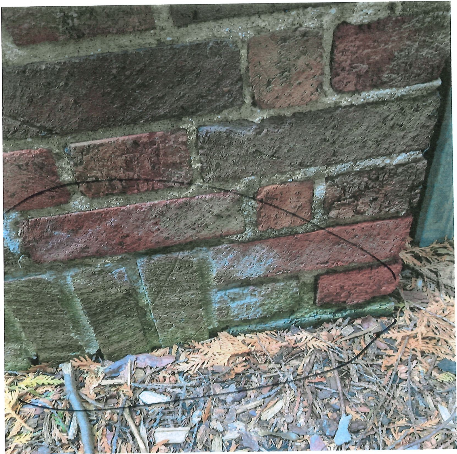
⑨ Tuckpointing/brick maintenance
