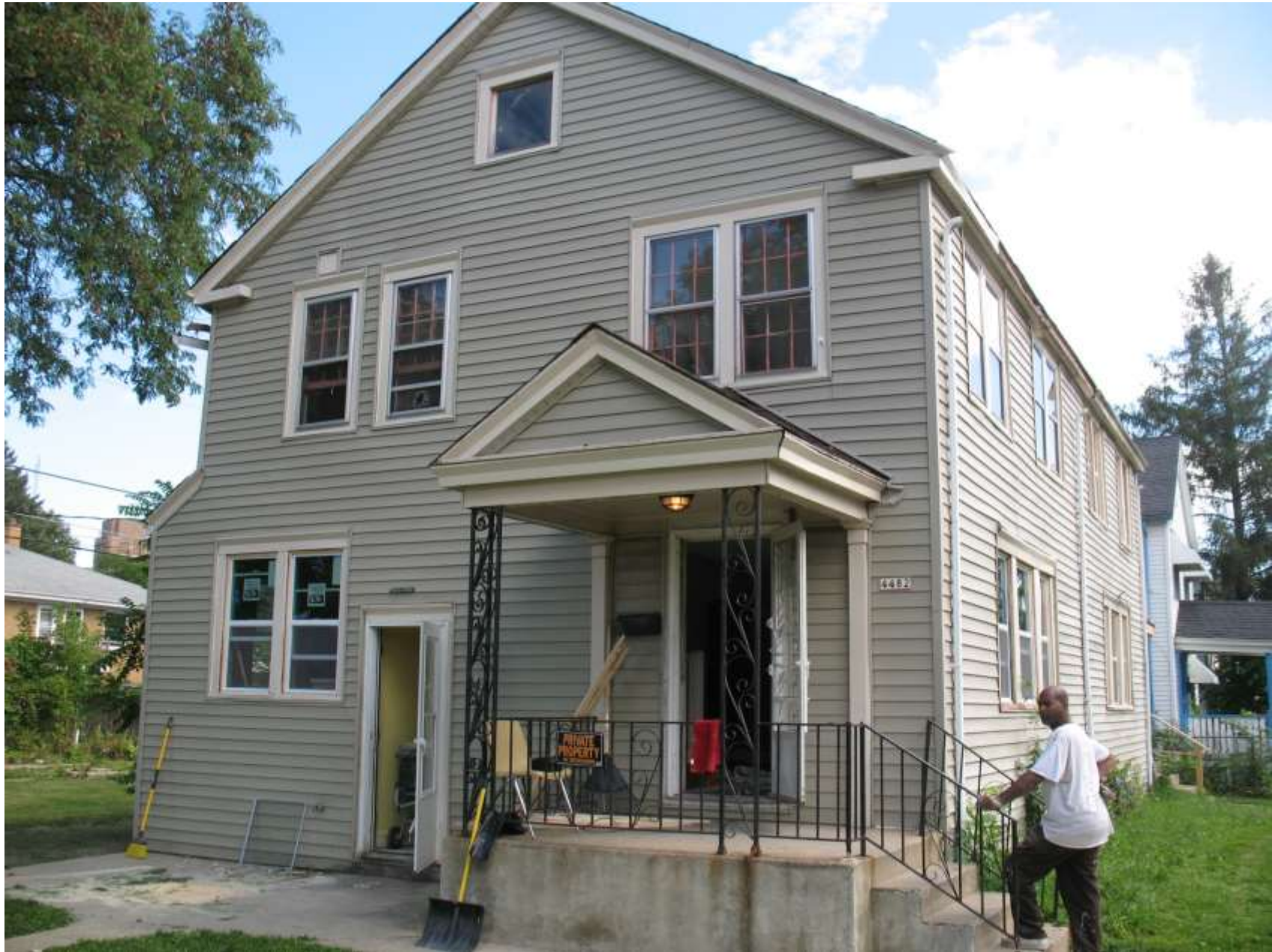
Work in progress, see bottom left.
