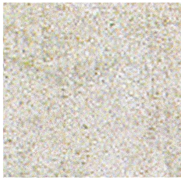
CAST IN PLACE CONCRETE
