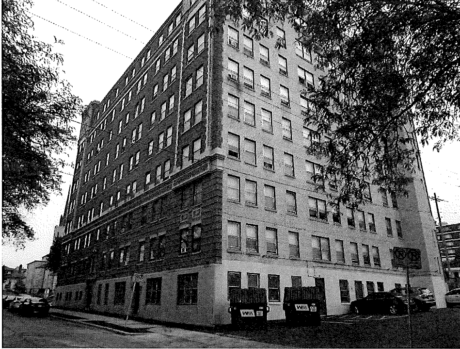
View looking northeast from N. 31 st St.
