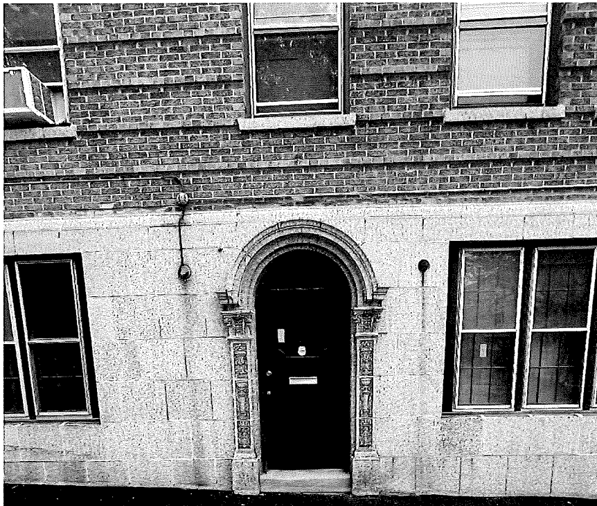
Service entrance on N. 31 st St.
