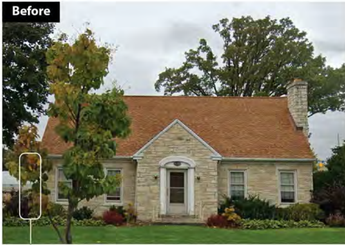
Bay window removed on south side. Not visible in this photo.
