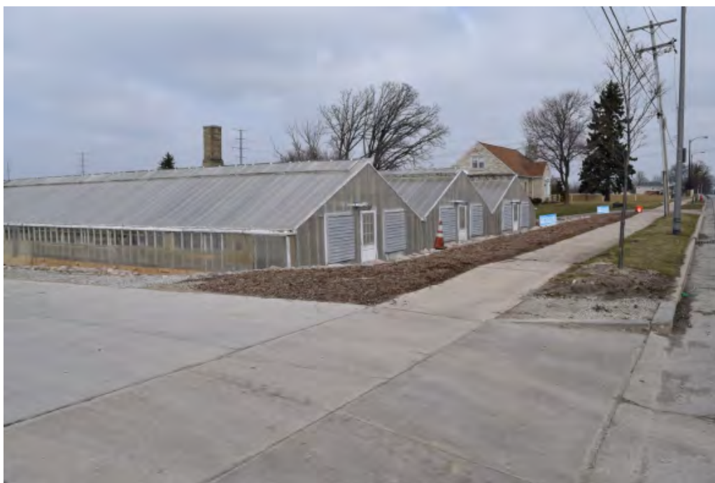
BUILDINGS 3 & 1 – looking north from sidewalk along property line
