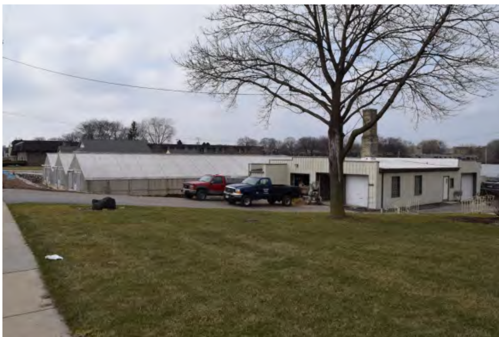
BUILDINGS 2 & 3 – looking southwest from sidewalk
