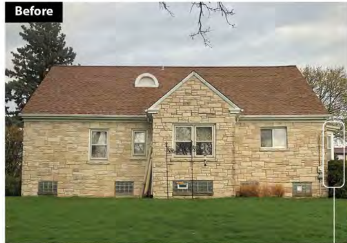
Bay window removed on south side.
