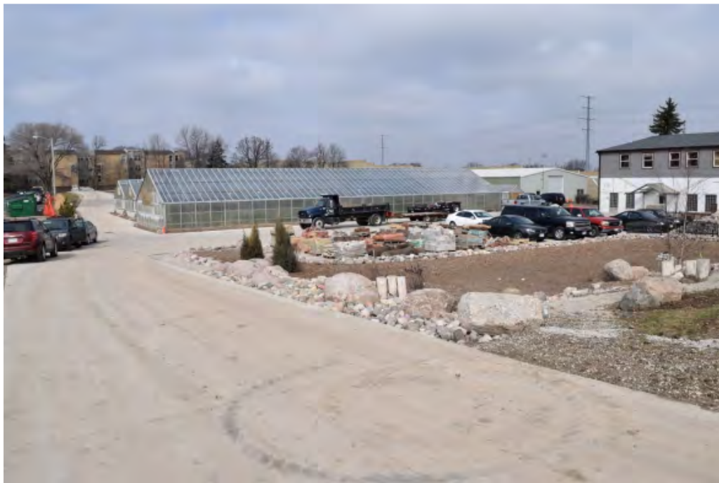
BUILDINGS 7, 6, & 5 – looking northwest from center of south property line
