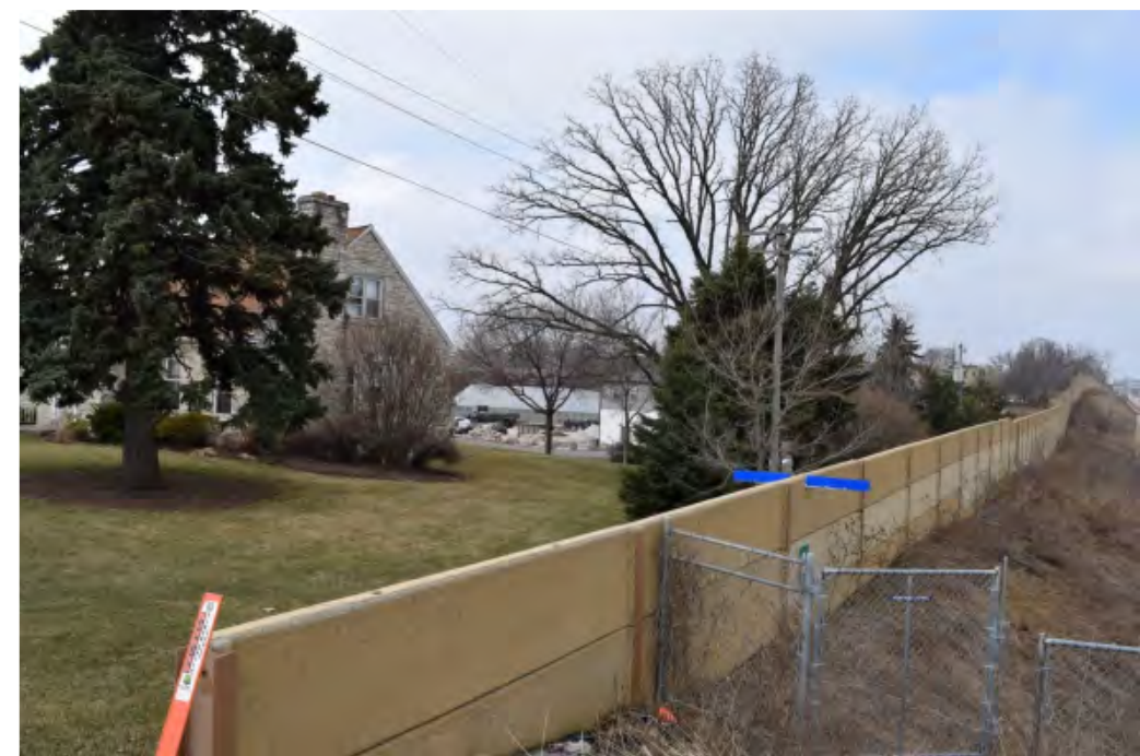
BUILDING 1 – looking west from sidewalk along property line
