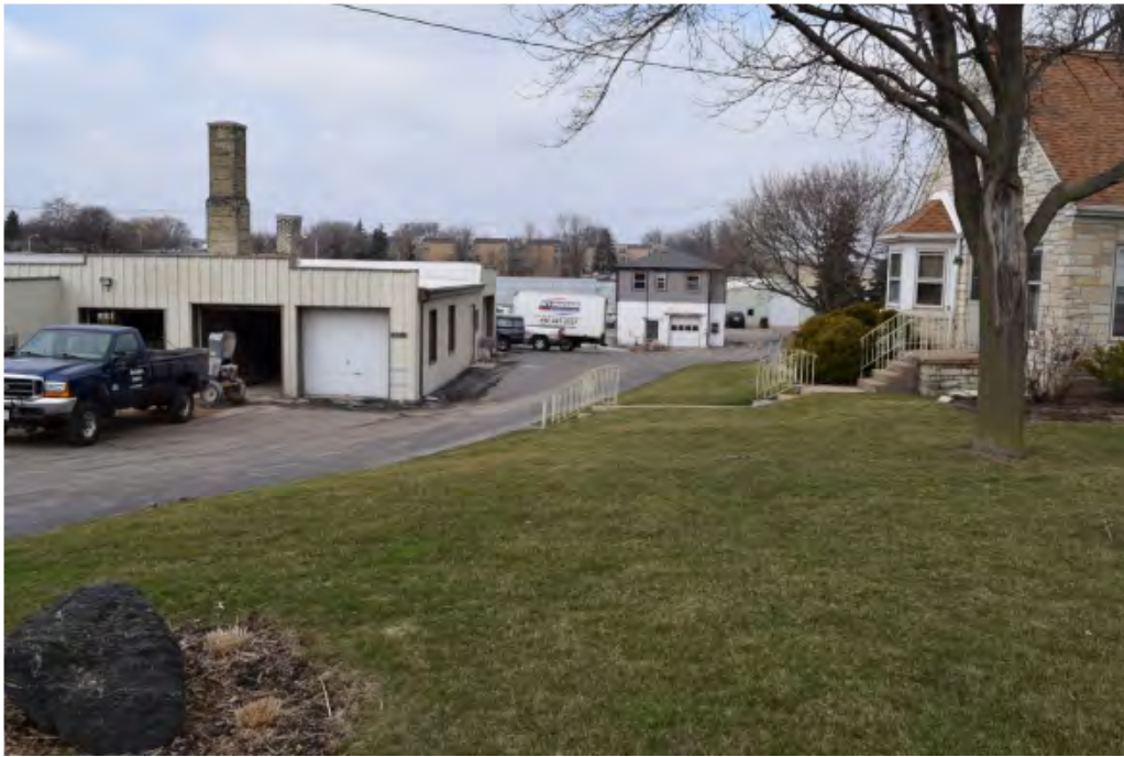
BUILDING 2 – looking west from sidewalk
