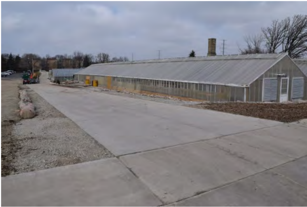
BUILDING 3 – looking west from sidewalk along property line
