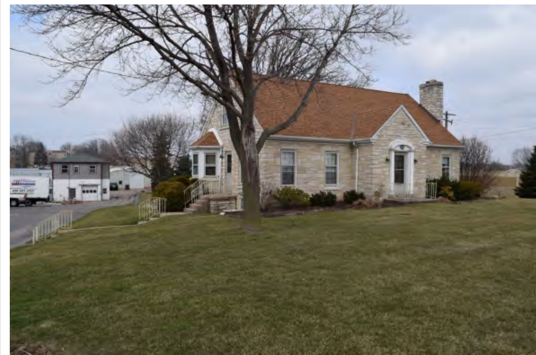
BUILDING 1 – looking west from sidewalk
