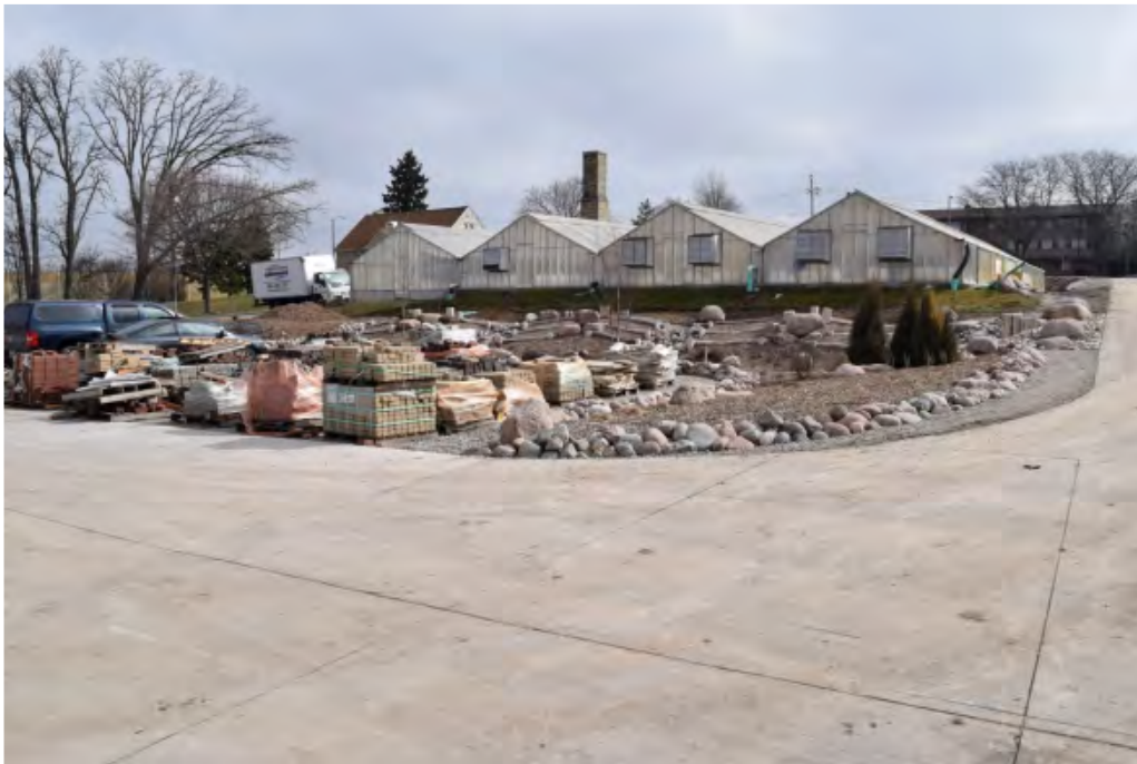
BUILDING 3 – looking northeast from center of south property line
