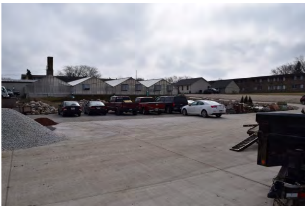
BUILDINGS 2 & 3 – looking east from center of property
