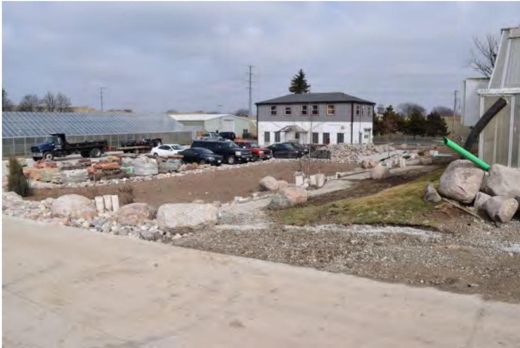
BUILDINGS 7, 6, 5, & 3 – looking north from center of south property line
