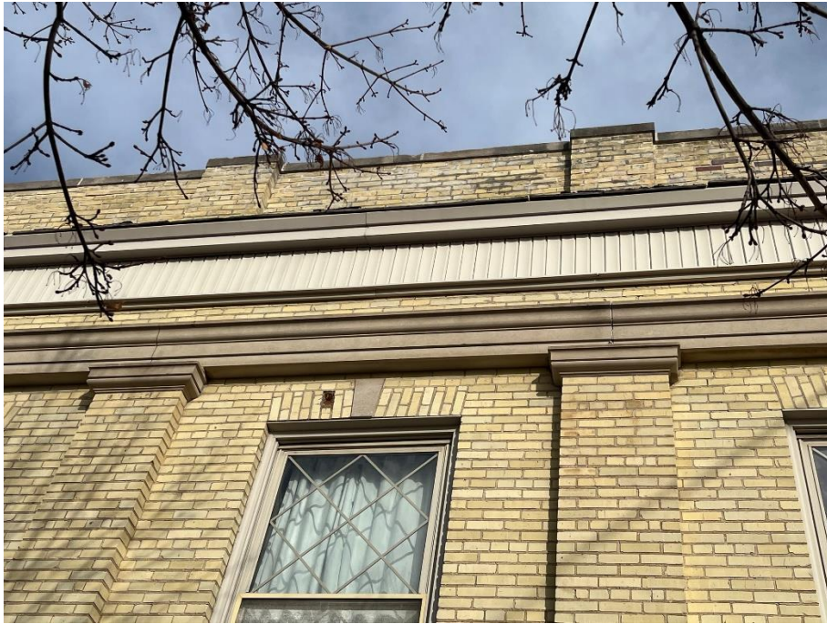
Rear parapet tuck pointing
