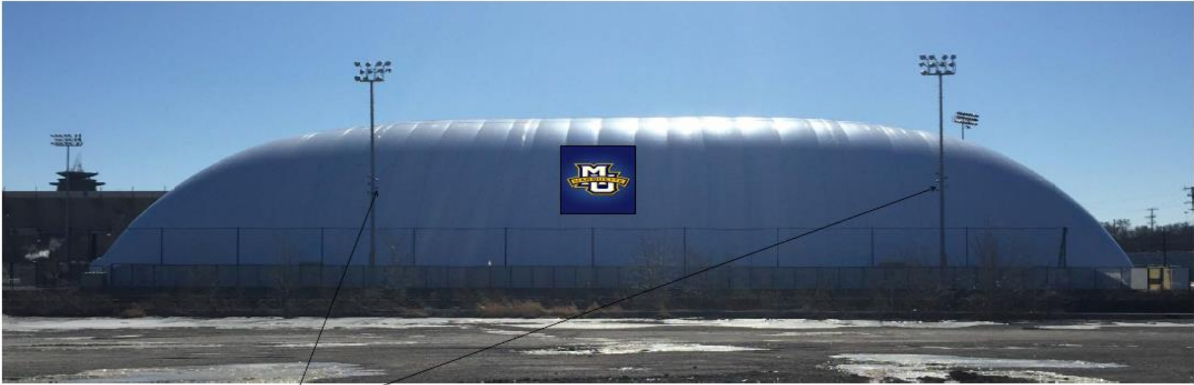
Spotlight Fixture For Evening Illumination Fixed to Light Poles
